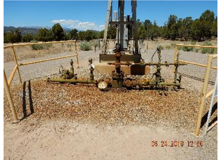
Photo 8: Impacted soil and gravel around 1B wellhead.
