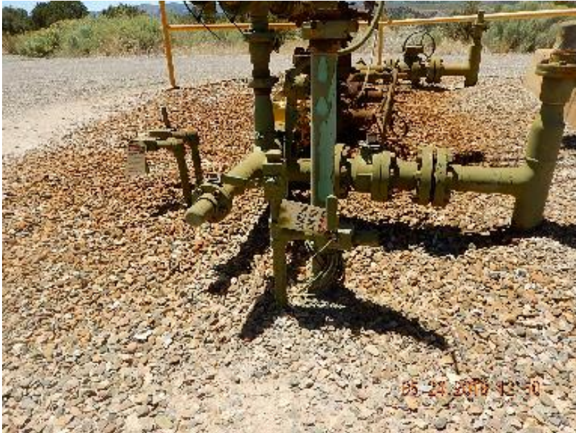
Photo 5: Unused steel 1" riser at 1B.
