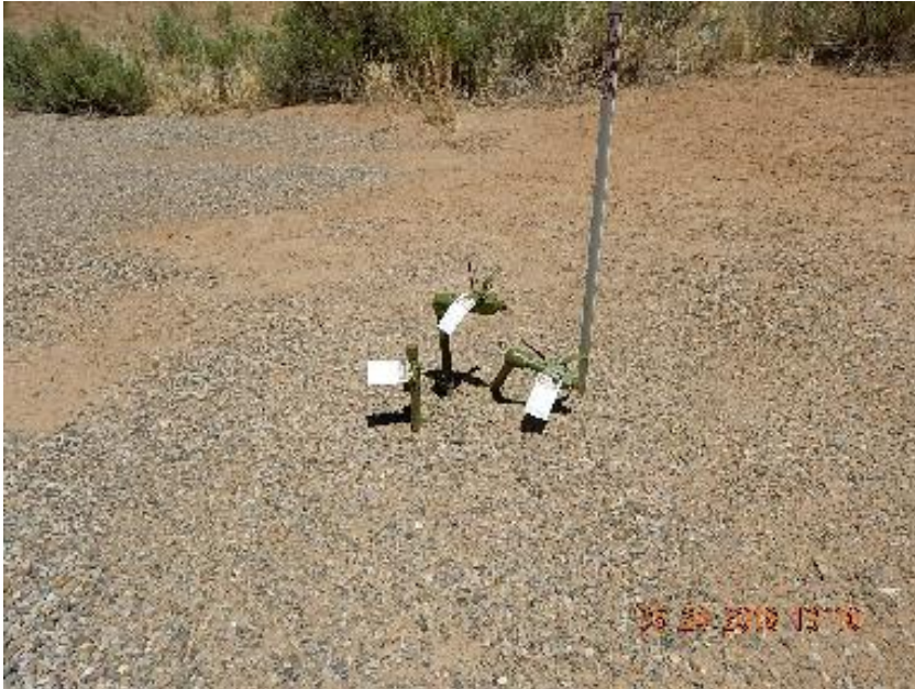
Photo 7: Unused steel 1" risers on E side of separator.
