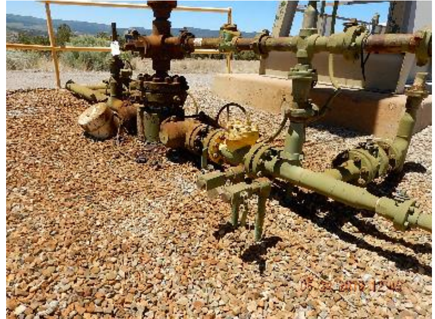
Photo 4: Unused steel 1" risers at 1B.
