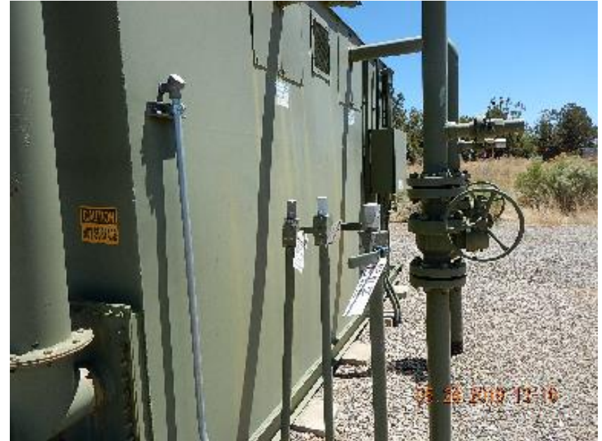
Photo 6: Unused steel 1" risers on W side of separator.
