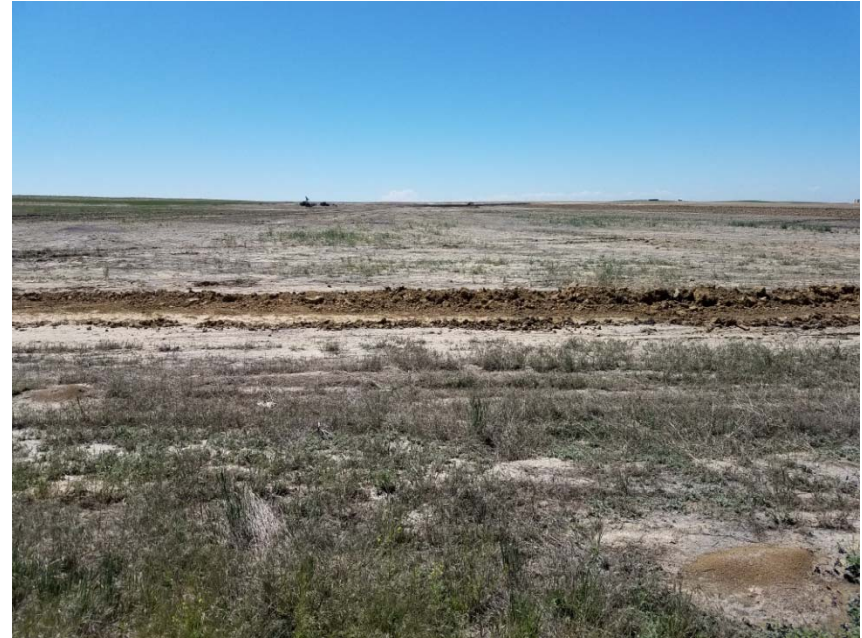
Photo 2 – From north end of Krier 4 Land Application Area at Carlson 22-1 tank battery looking south. Soil has been roughened in the middle of photo to aid in prevention of offsite liquid migration.
