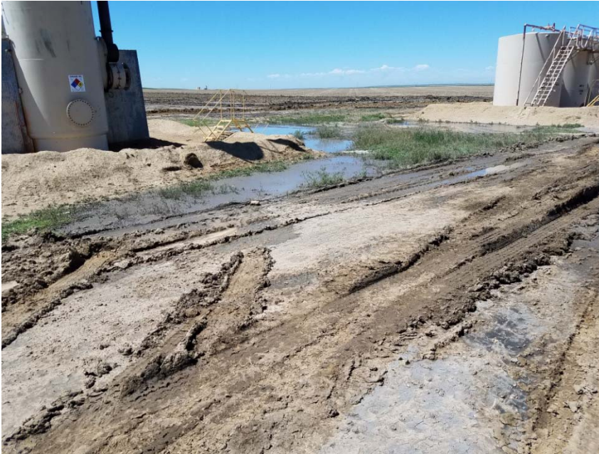
Photo 5 – On the Carlson 22-1 tank battery, impacted by drilling fluid runoff from the Krier 4 land application site.
