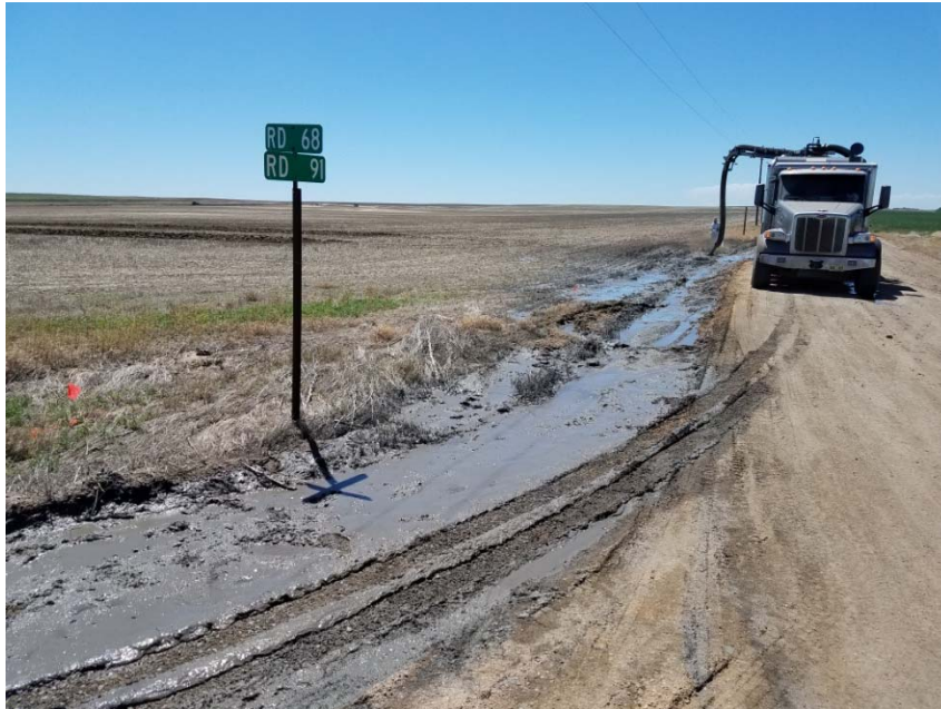
Photo 9 – Photo at Weld County Roads 68 and 91, looking south. Removal of drilling fluids is underway.
