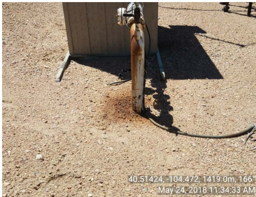
Photo 3: Stained soil at meter run
