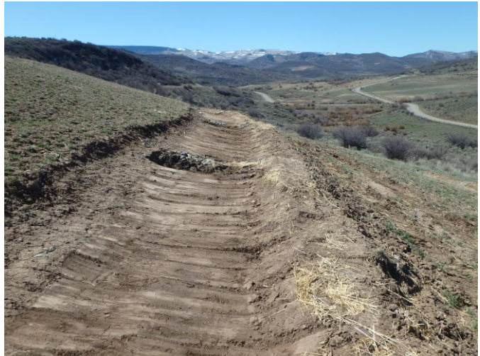
Water Bar on BCU 12B after Maintenance
