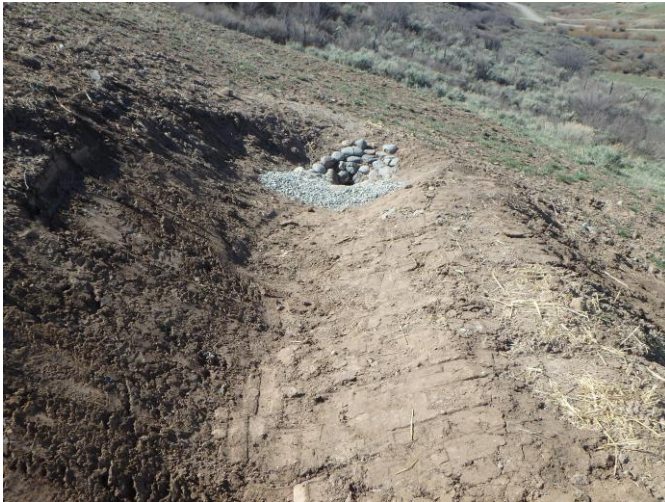
Breach in Water Bar on BCU 12B after Repairs
