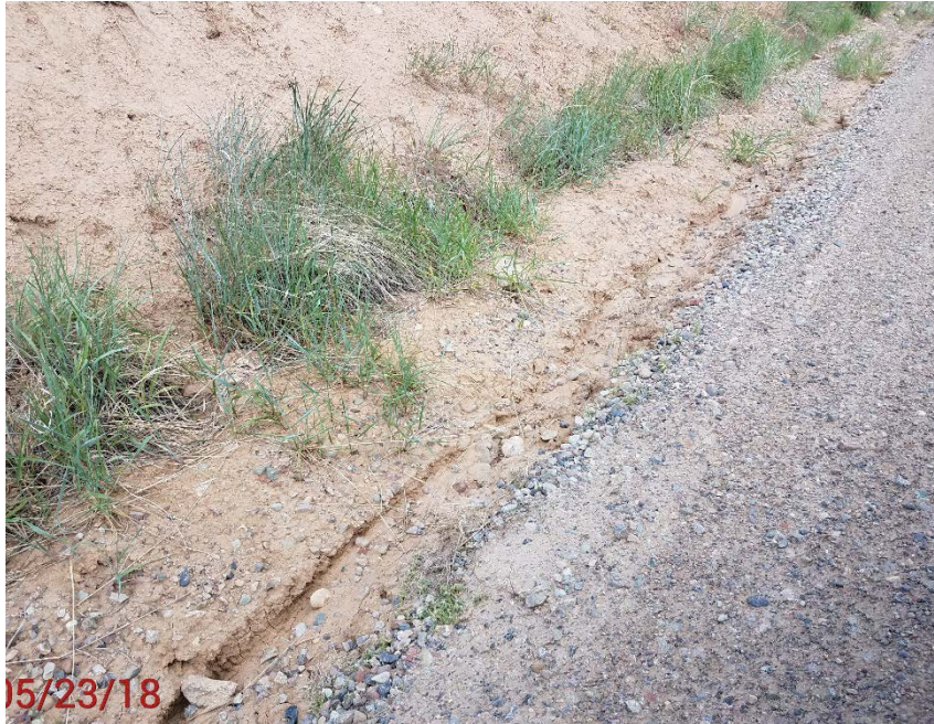
Location Photo #11, Ditch erosion along side of road on east side near curve
