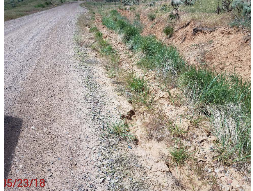
Location Photo #8 , Ditch erosion along side of road on east side. Looking down hill
