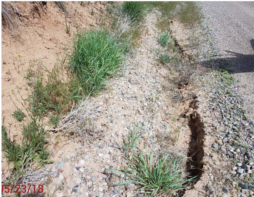
Location Photo #9, Ditch erosion along side of road on West side. Looking down hill
