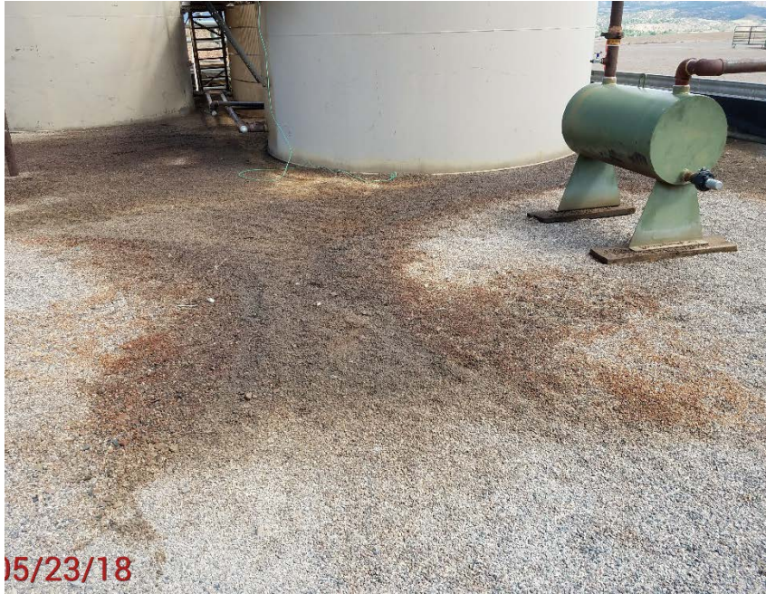
Location Photo #5, stained material in battery containment
