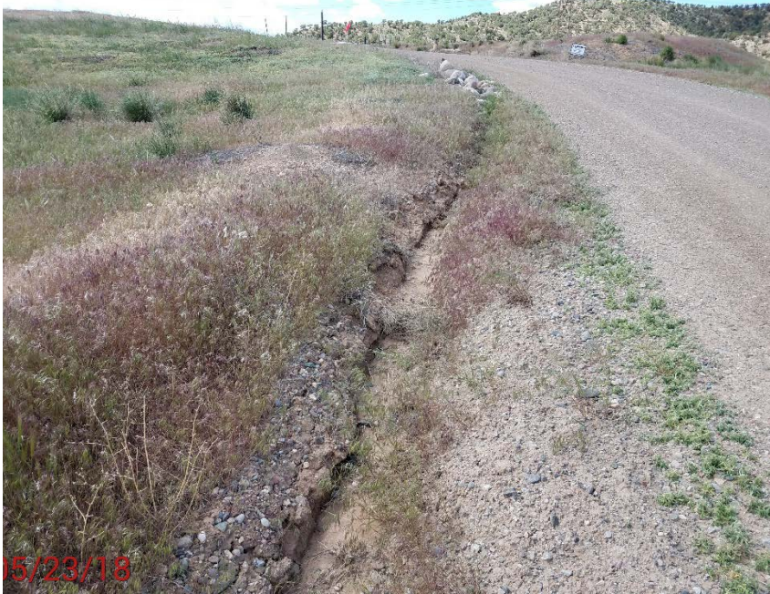
Location Photo #7, Ditch erosion along side of road on east side
