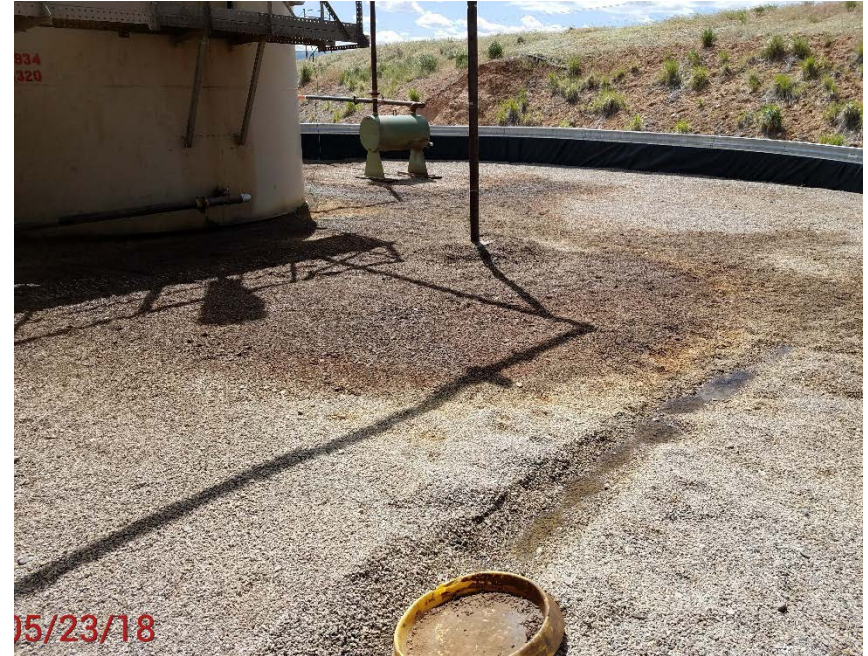
Location Photo #4, stained material in battery containment
