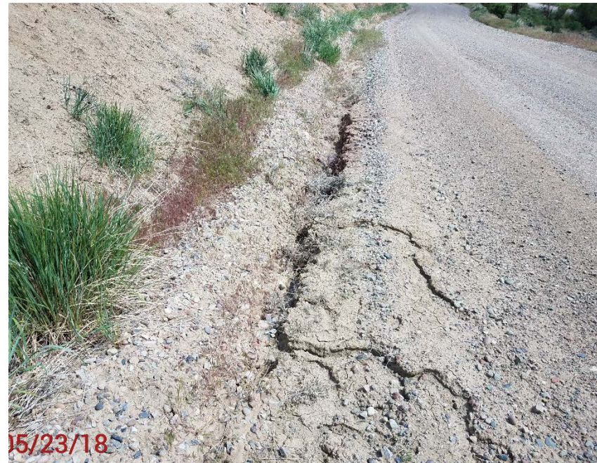
Location Photo #10, Ditch erosion along side of road on West side. Looking downhill
