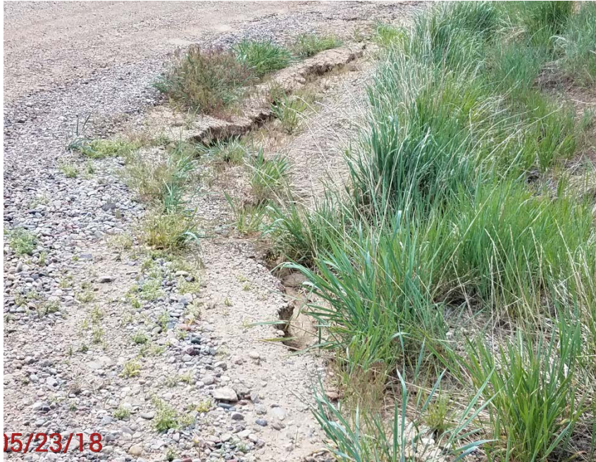
Location Photo #13, Ditch erosion along side of road on east side at the curve
