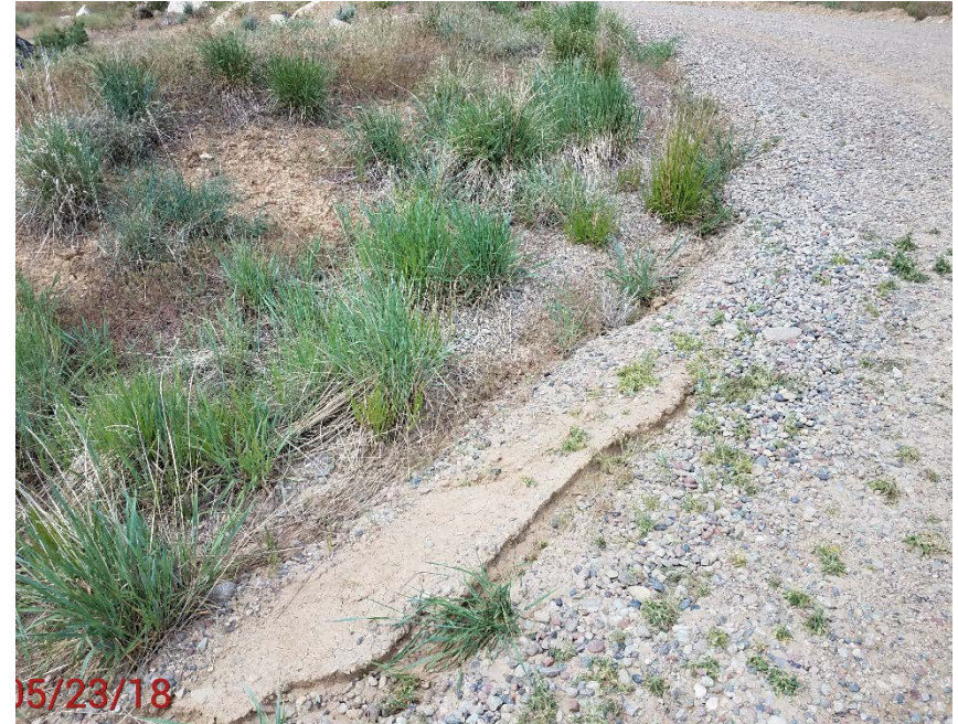
Location Photo #14, Ditch erosion along side of road on east side at the curve
