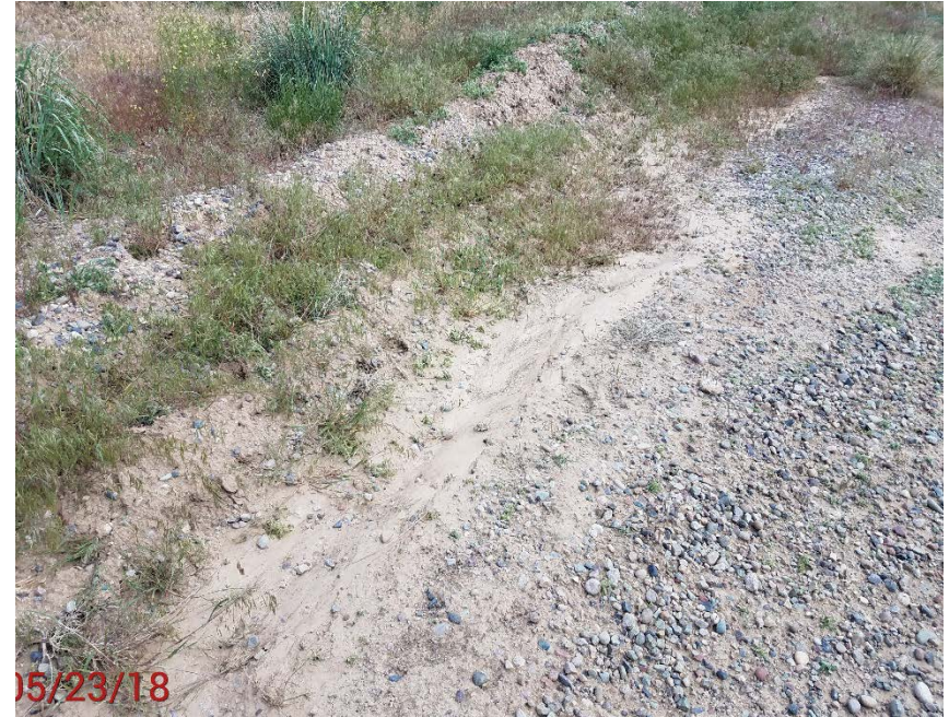
Location Photo #12, Ditch erosion along side of road on east side near curve
