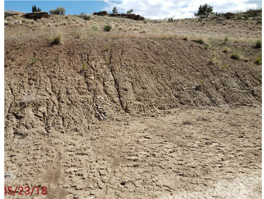
Location Photo #7, Slope erosion behind tank battery
