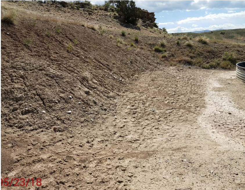
Location Photo #6, soil build up from slope erosion.
