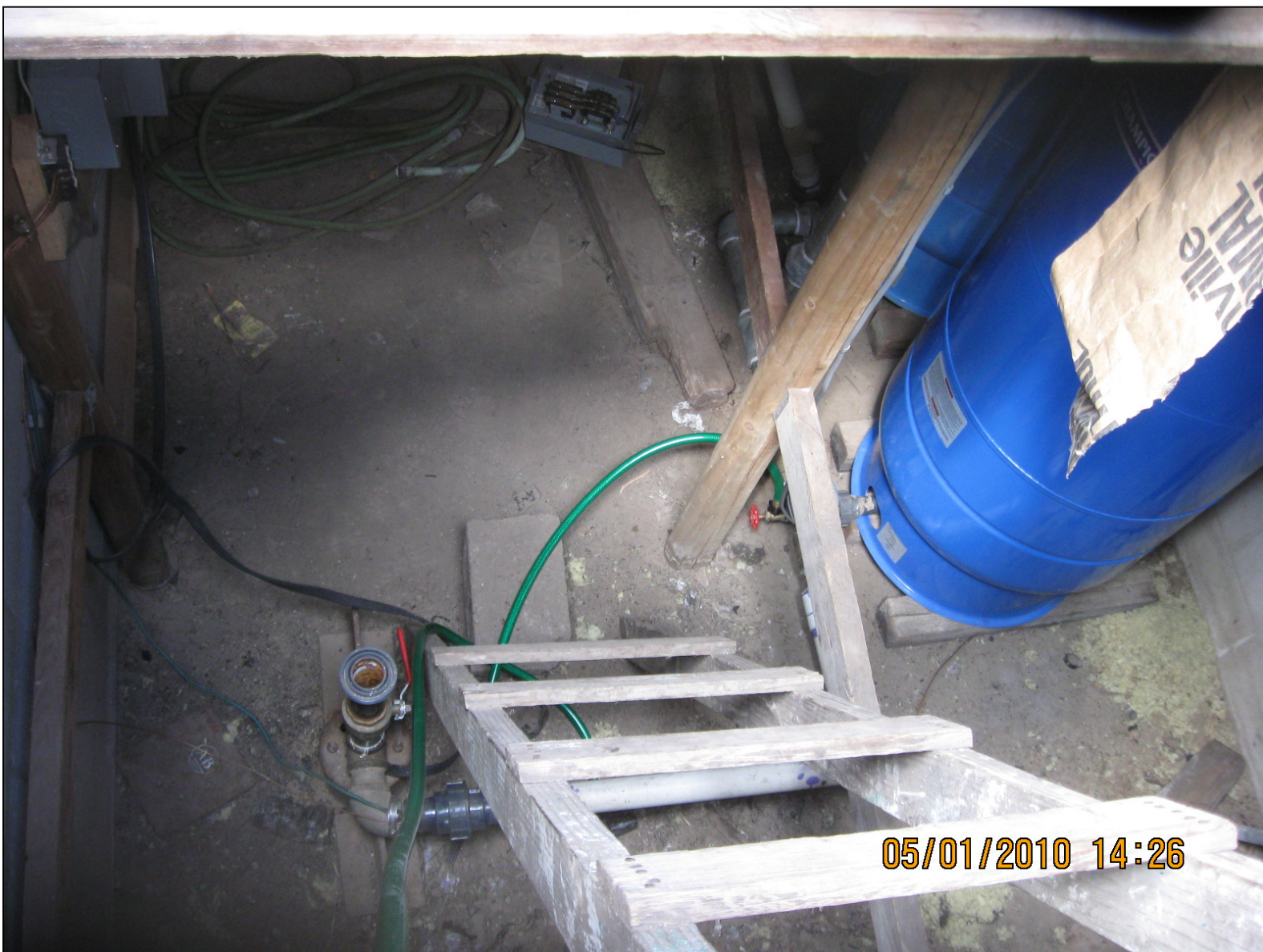
Figure 9. Photograph of pressure tank in Mr. William's dugout outside his house. Well water with high dissolved methane concentration (~9 ppm) is fed directly into the tank without venting. The methane will exolve from the water and build-up to explosive levels (5% by volume) in the tank and then be released into the residence when taps are turned on.
