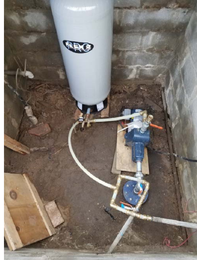
Photo 2 –View of water well vault for water well permit no. 276778 with new well seal, pump/motor and pressure tank.
