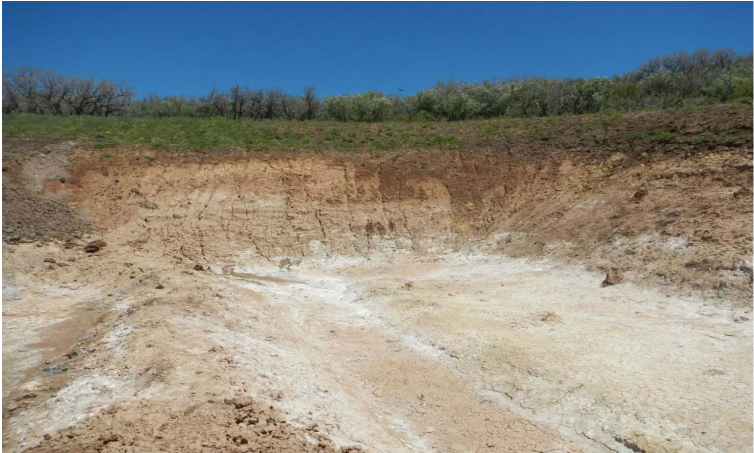
Photo#1: Southeast section of cut slope where stabilization is needed.
