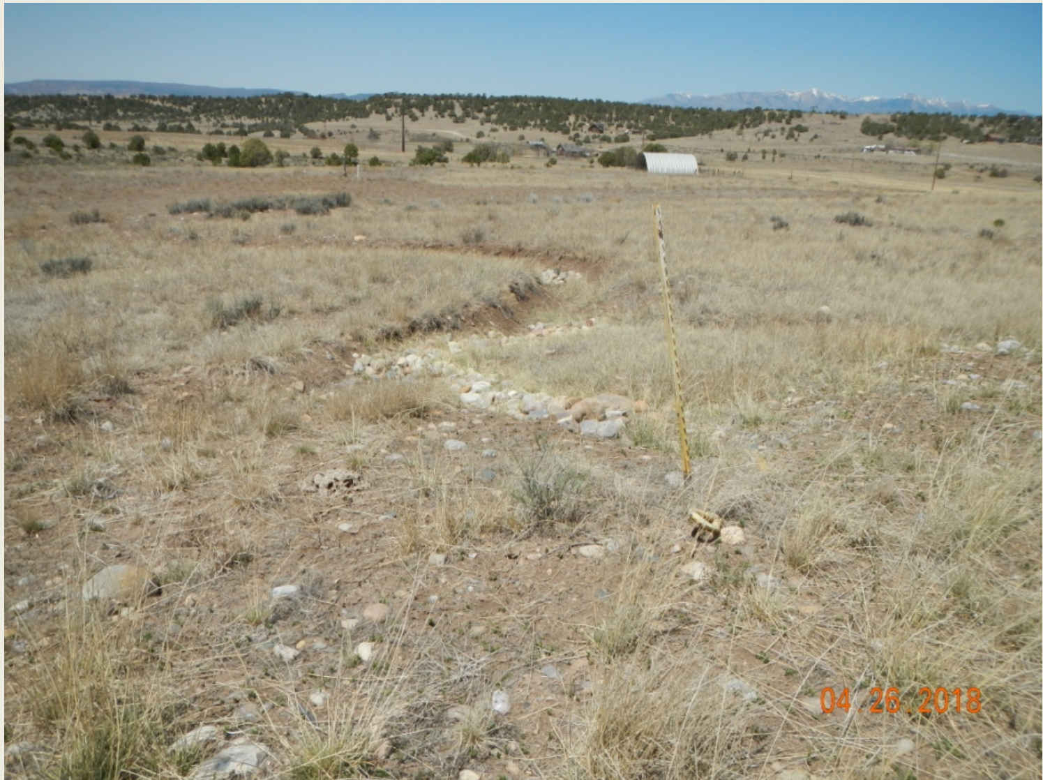
Photo 5. View of stormwater controls within the western portion of the project area appear to be added after erosional channel was formed.
