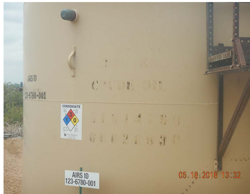
Photo 2: Faded tank stenciling on condensate tank
