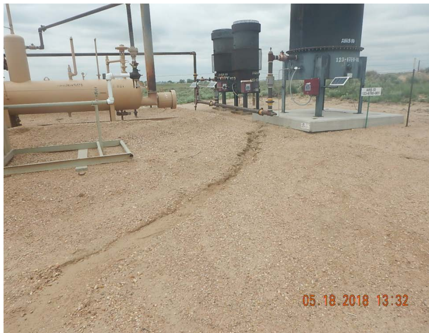
Photo 3: Stormwater erosion SW of ECD, looking NE.
