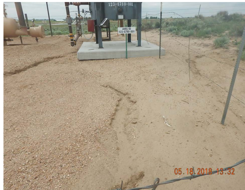
Photo 4: Stormwater erosion S of ECD, looking N.
