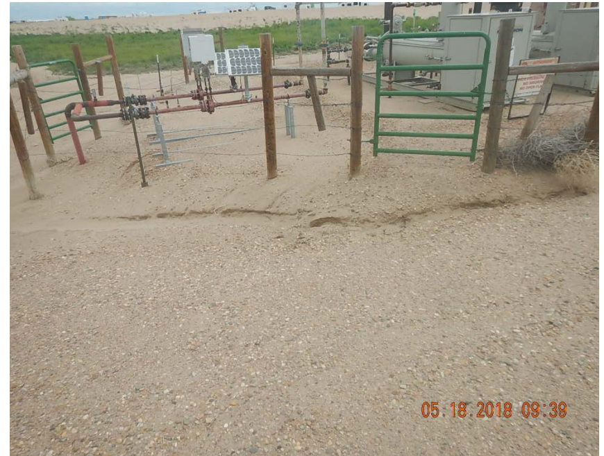
Photo 4: Stormwater erosion at SW side of separators
