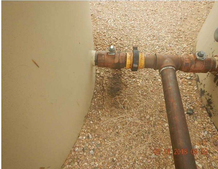
Photo 5: Stained soil at fitting.
