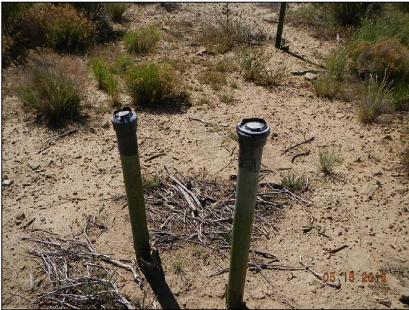
Photo 3. Disconnected risers.
