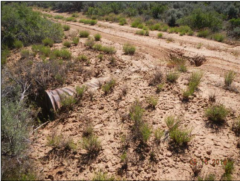
Photo 5. Damaged culvert.
