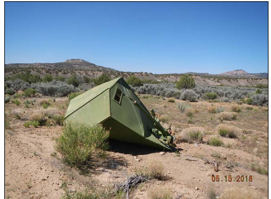
Photo 2. Disconnected meter house.
