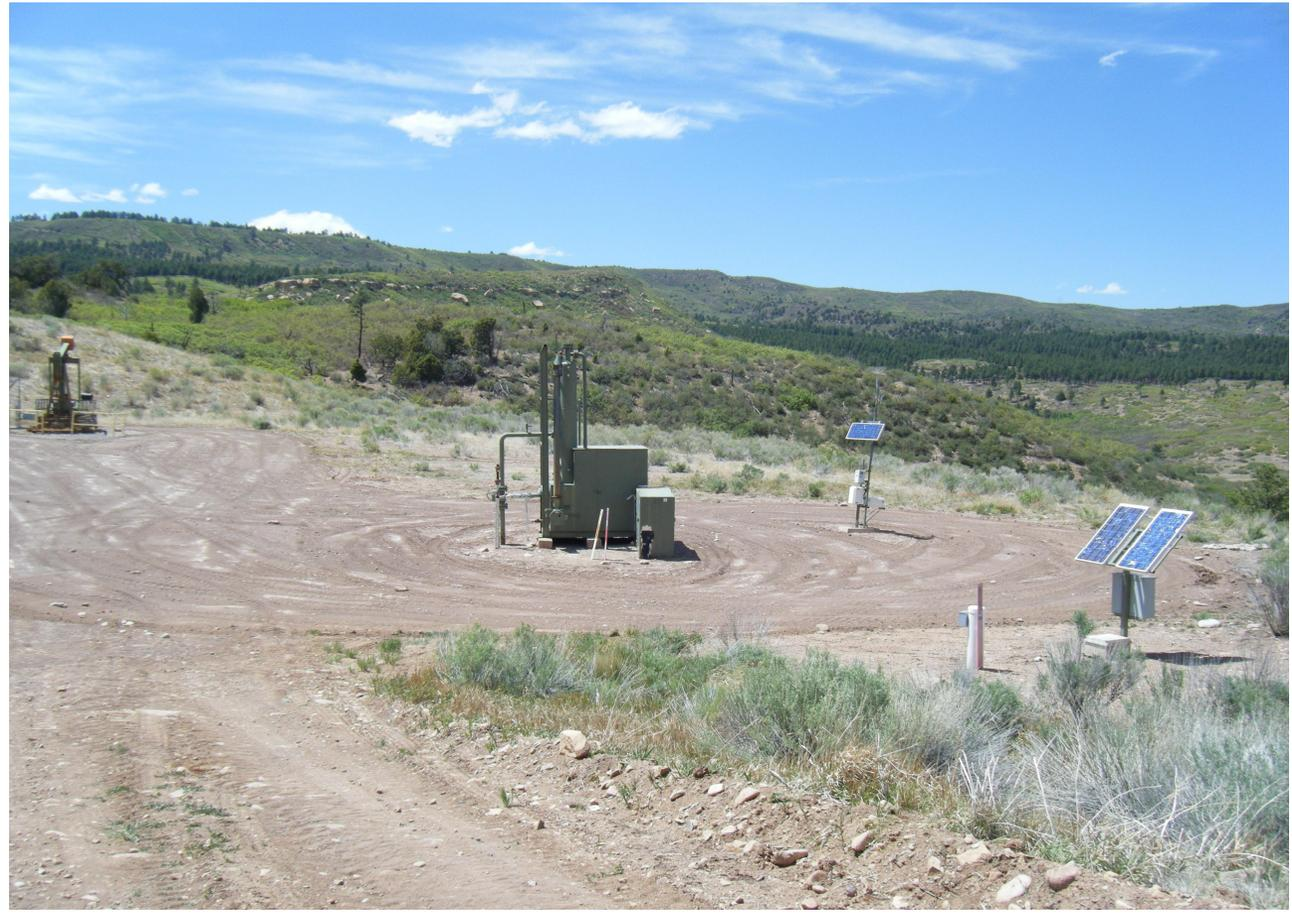
Corrective action taken for Photo 6 & 7 from inspection report. Stormwater management controls have been established to stabilize erosion in the Northeast portion of project area.
