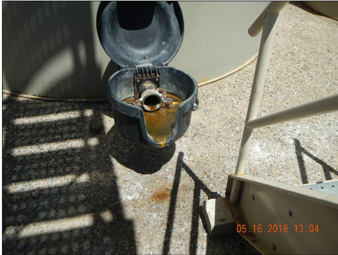
Spill pan full and dripping inside of secondary containment.
