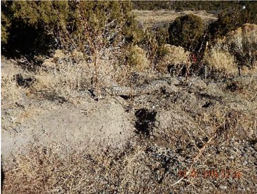
Photo 11: Breach in berm and undercut straw waddle previous inspection.
