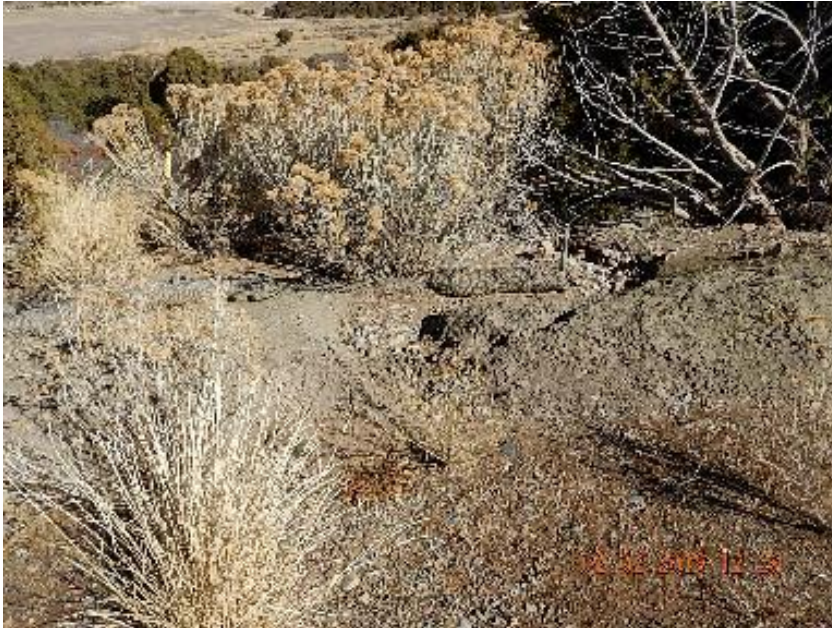
Photo 9: Breach in berm NE corner with erosion channel in background previous inspection.
