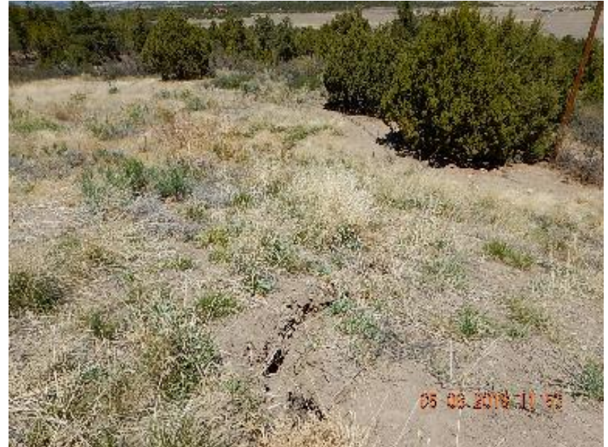
Photo 14: Erosion channel on fill slope. Corrective action not completed.
