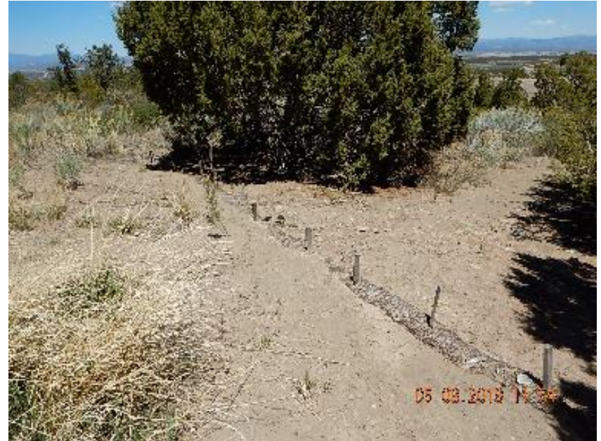
Photo 20: Full waddles at bottom of fill slope.
