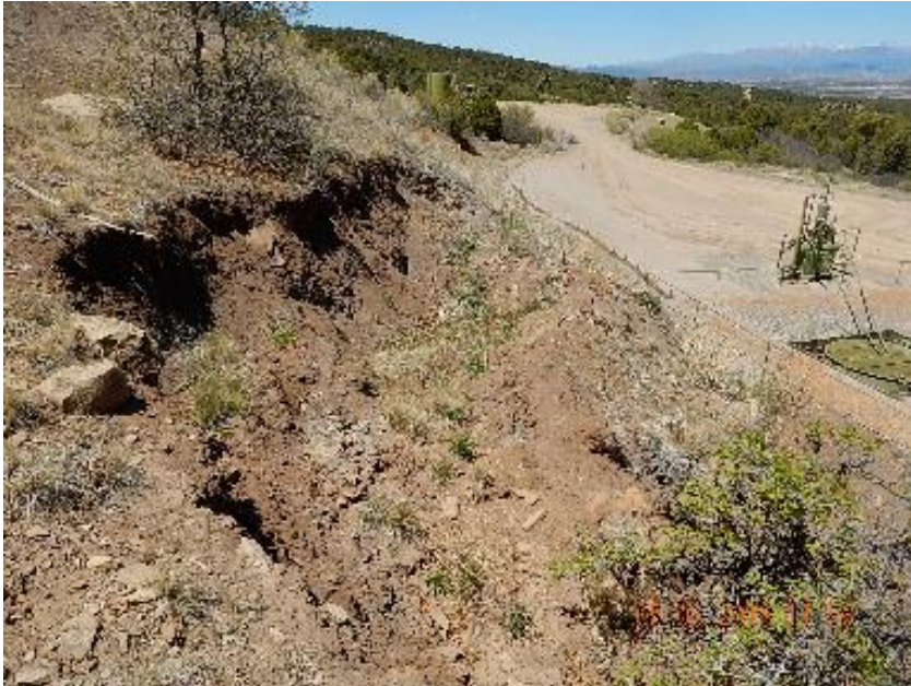
Photo 19: View at top of cut slope slide area.
