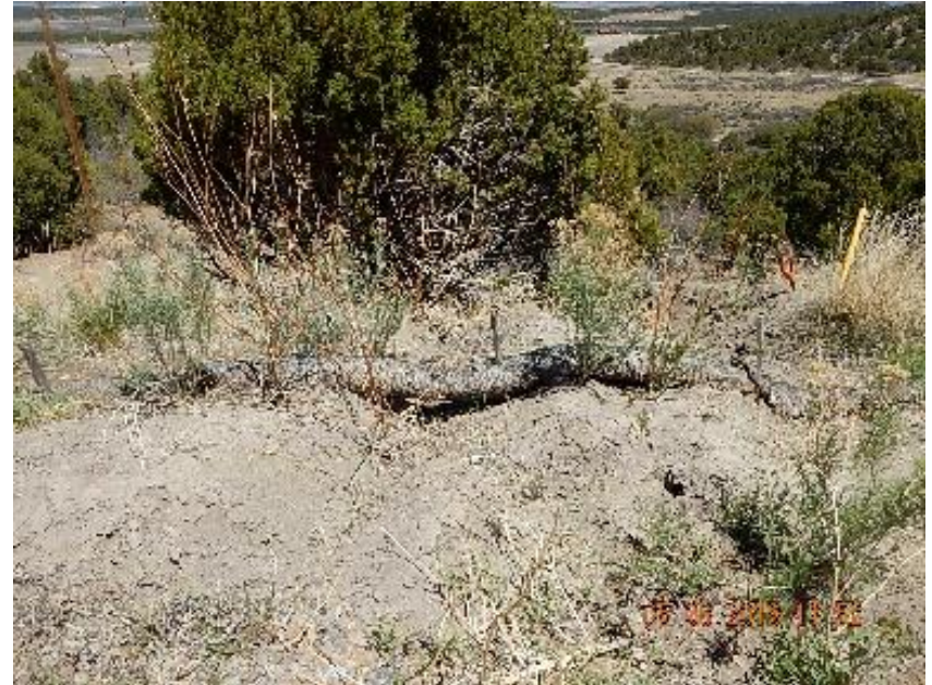
Photo 12: Breach in berm and undercut straw waddle. Corrective action not completed.
