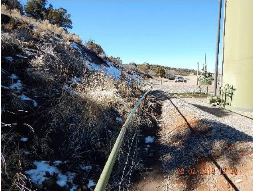
Photo 17: Slide pushing into tank battery fencing previous inspection.
