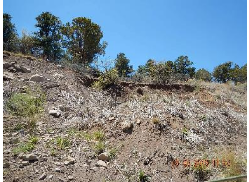
Photo 16: Cut slope slide area behind tank battery. Corrective action not completed.
