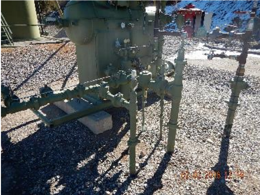
Photo 7: Flow lines at separator previous inspection.
