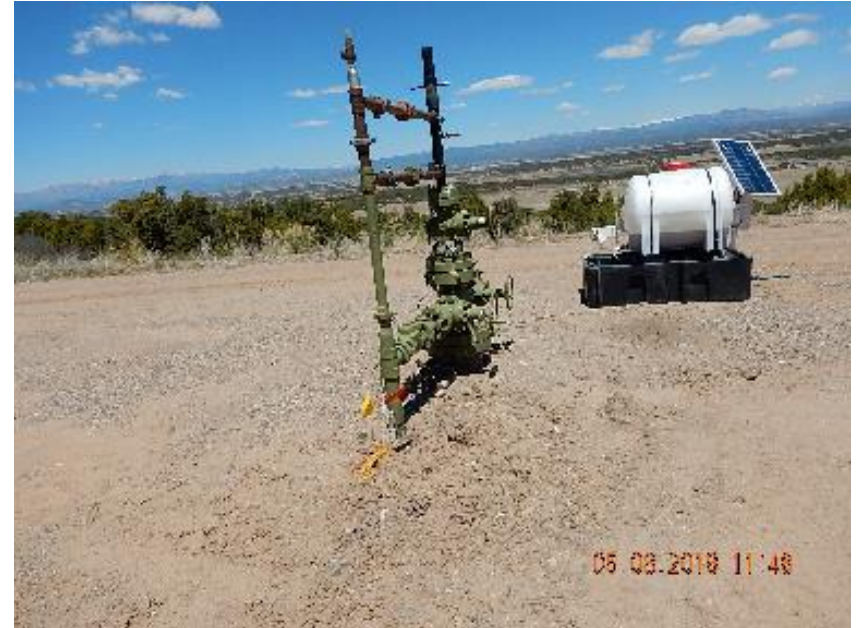
Photo 6: Wellhead after risers abandoned.
