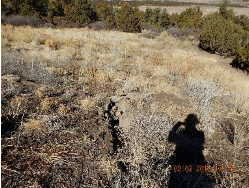
Photo 13: Erosion channel on fill slope.
