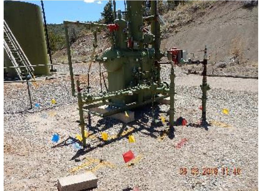
Photo 8: Separator after flow lines abandoned.
