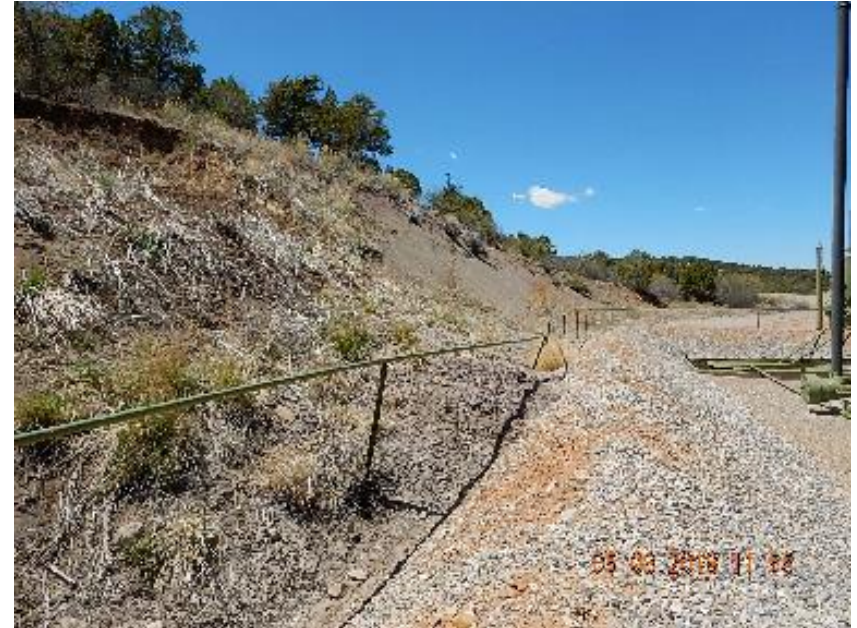
Photo 18: Slide pushing into tank battery fencing. Corrective action not completed.
