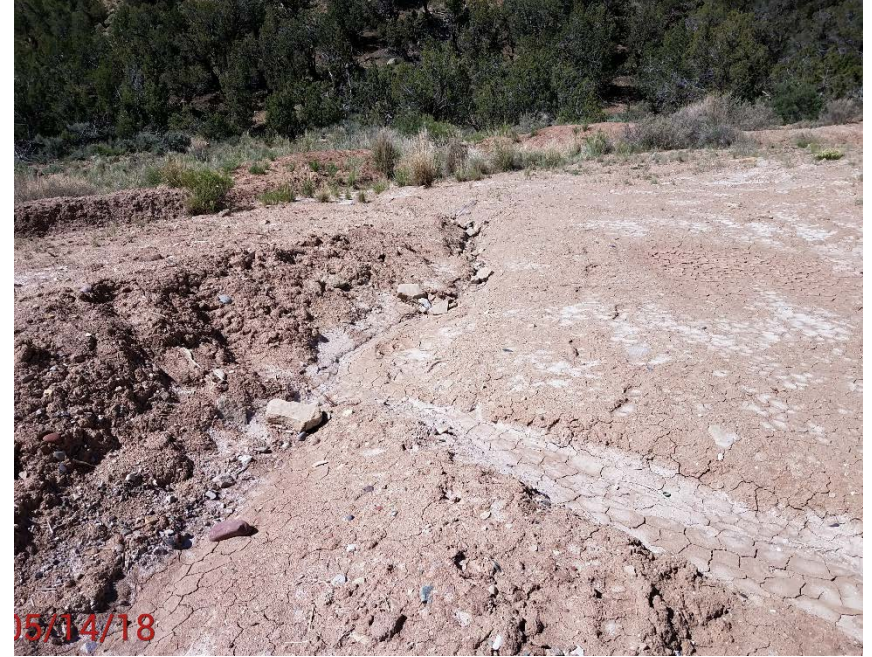
Location Photo #2, Erosion on South west end of location
