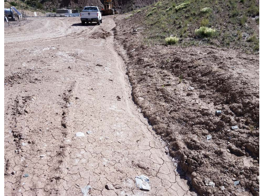
Location Photo #4, ditch along south side of location, storm water issue
