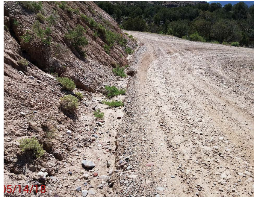
Location Photo #14, Ditch Erosion along access road near the Y
