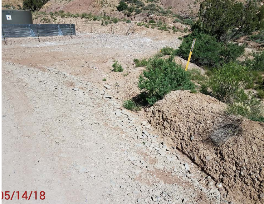
Location Photo #11, Erosion near end of location by access road
