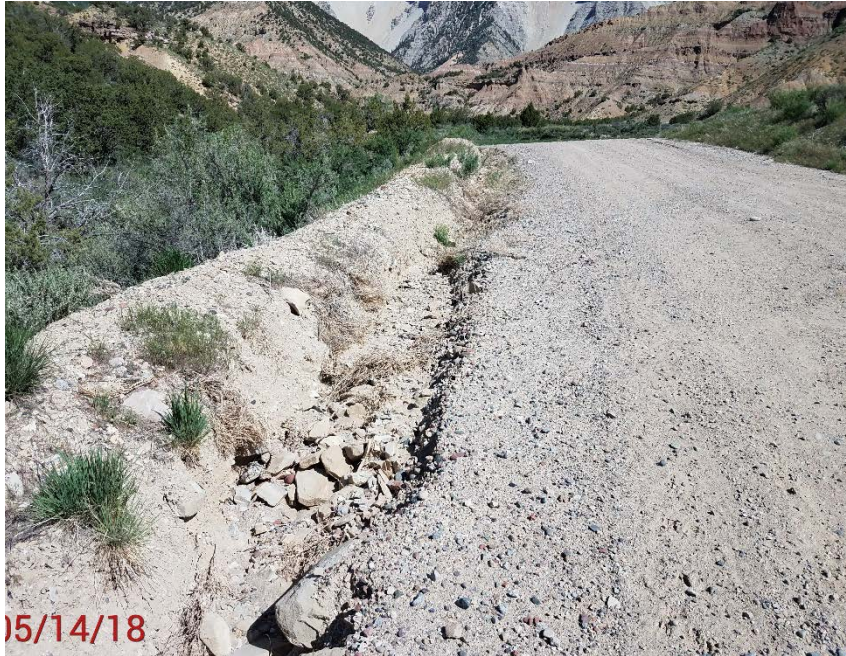
Location Photo #3, Erosion on the west side of the access road, near location. Looking uphill
