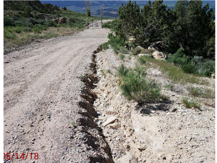
Location Photo #4, Erosion on the side of the access road looking South downhill .
