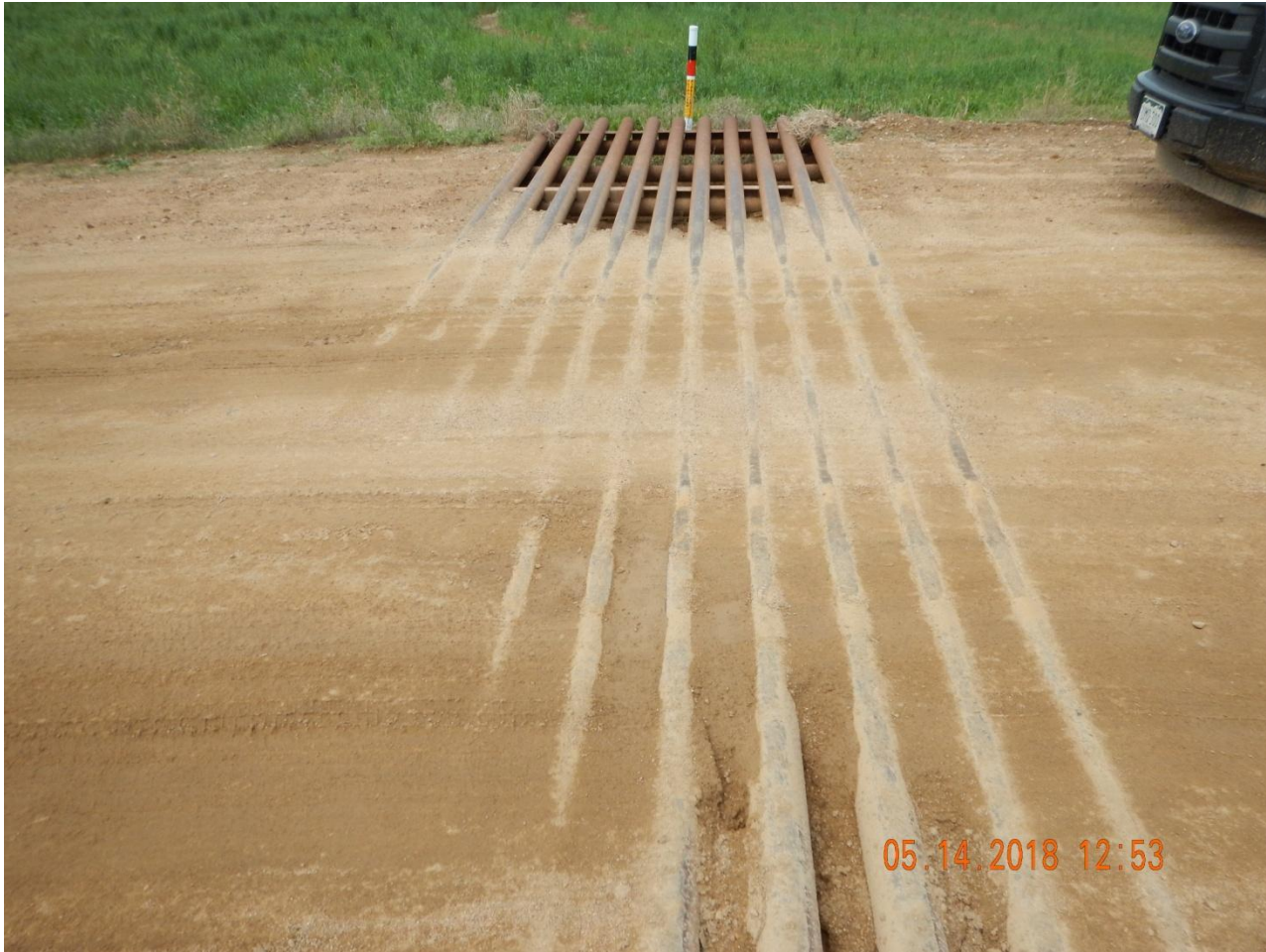
Photo 4. Photo taken from a portion of the access road. Cattle guard in need of maintenance. A similar inspection will be sent to the other Operator that also uses this BMP and access road. Both Operator's will need to coordinate to perform the required maintenance for this BMP.
