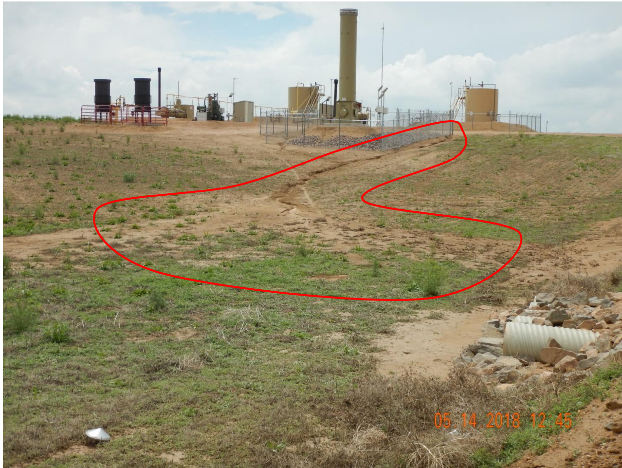
Photo 1. Photo taken of the northeast battery location, facing Southwest. Appears stormwater runoff from the battery location is causing rill erosion off location. There were no observed BMPs being implemented along the battery location to minimize erosion.
