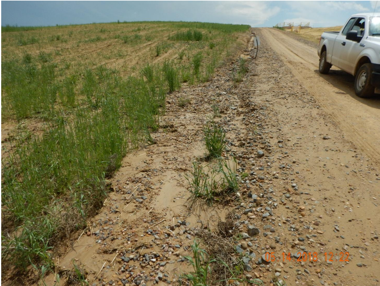
Photo 9. Photo taken from the east side of the access road, facing South. Photo illustrate sediment accumulation from rill erosion along the access road. There were no observed BMPs being implemented along the access road to minimize erosion.
