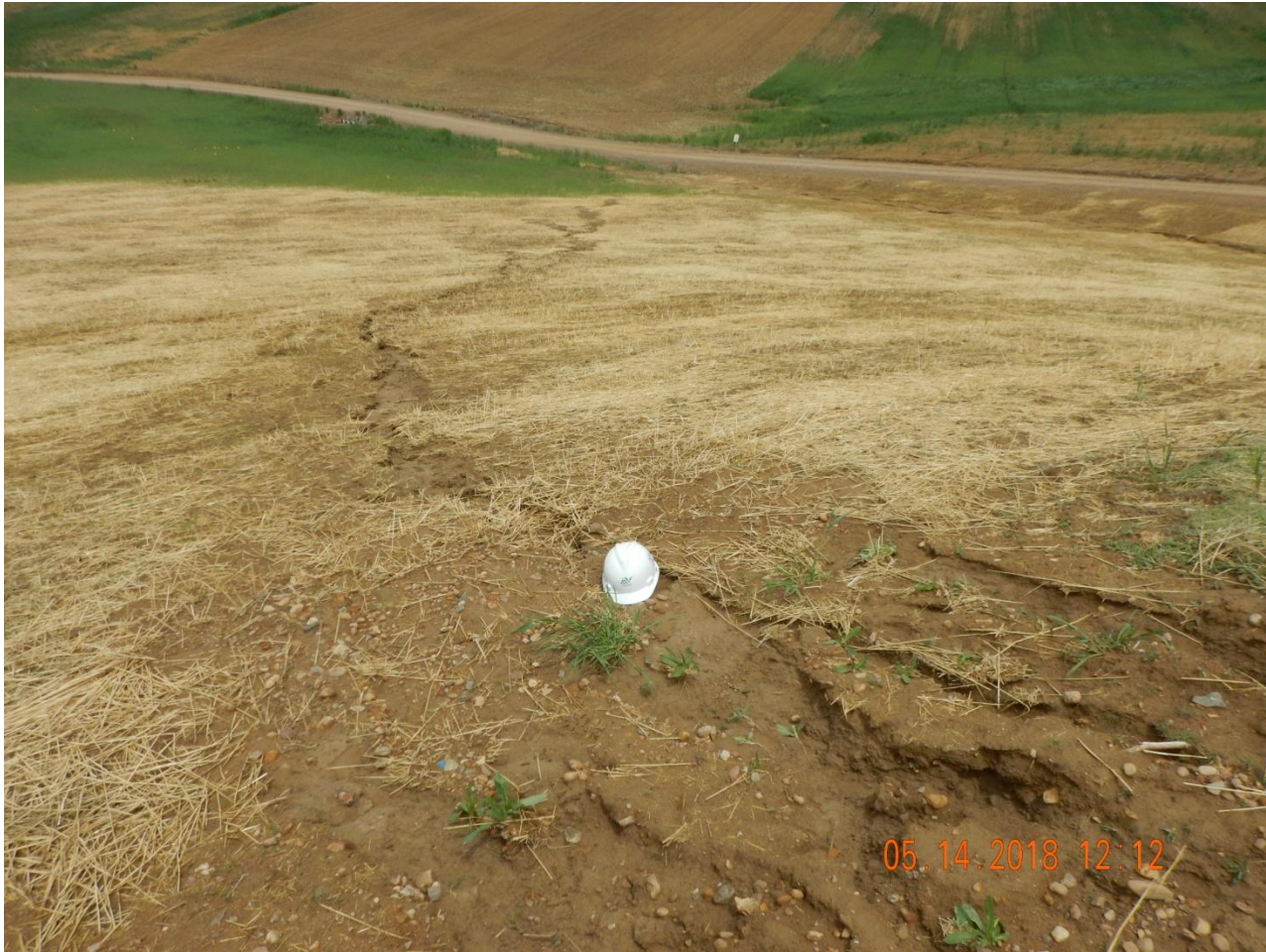
Photo 1. Photo taken of the northeast battery location, facing North. Appears stormwater runoff from the battery location is causing rill erosion off location and impacting interim areas.
