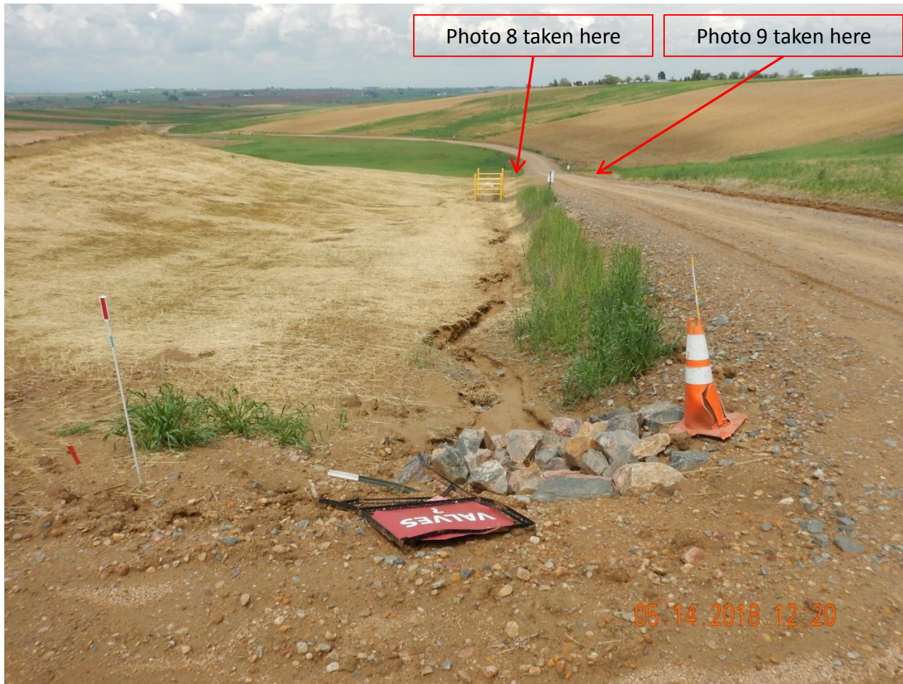
Photo 7. Photo taken from the entrance of the location, facing North. Appears the outlet protection BMP for the culvert is not properly functioning to minimize rill erosion along the eastern perimeter of the location.
