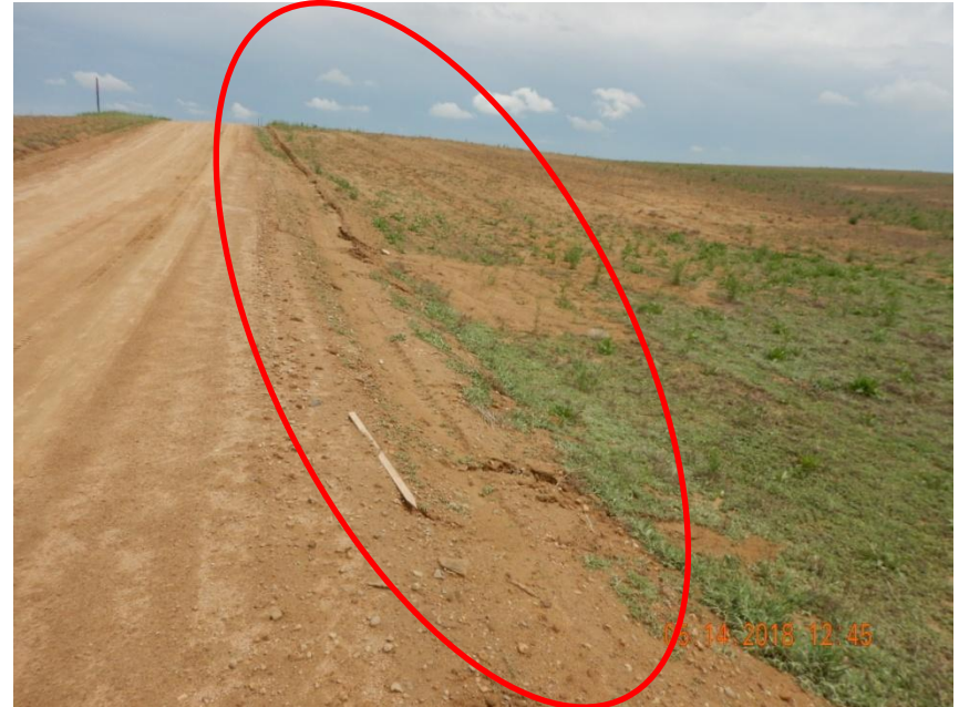
Photo 11. Photo taken from the opposite side of the access road, facing East. Rill erosion evident along portions of the access road. There were no observed BMPs being implemented along the access road to minimize erosion.
