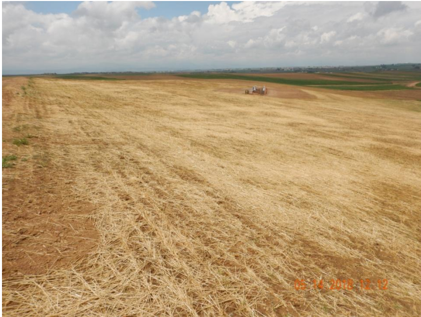
Photo 3. Photo taken of the northeast battery location, facing West. Appears the Operator has performed interim reclamation activities to reduce disturbance areas only needed for production operations, with the evidence of drilling rows and straw crimped mulch. Operator shall continue to monitor and manage this site until the location meets Rule 1003 standards.
