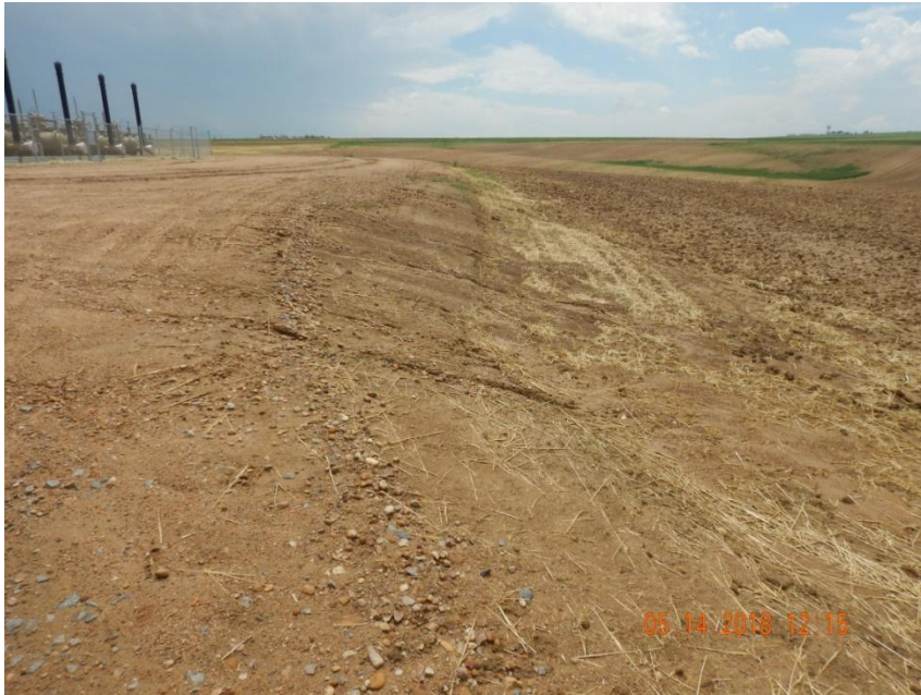
Photo 5. Photo taken of the northwest well location, facing South. Rill erosion evident along portions of the northeastern well location and along the access road.
