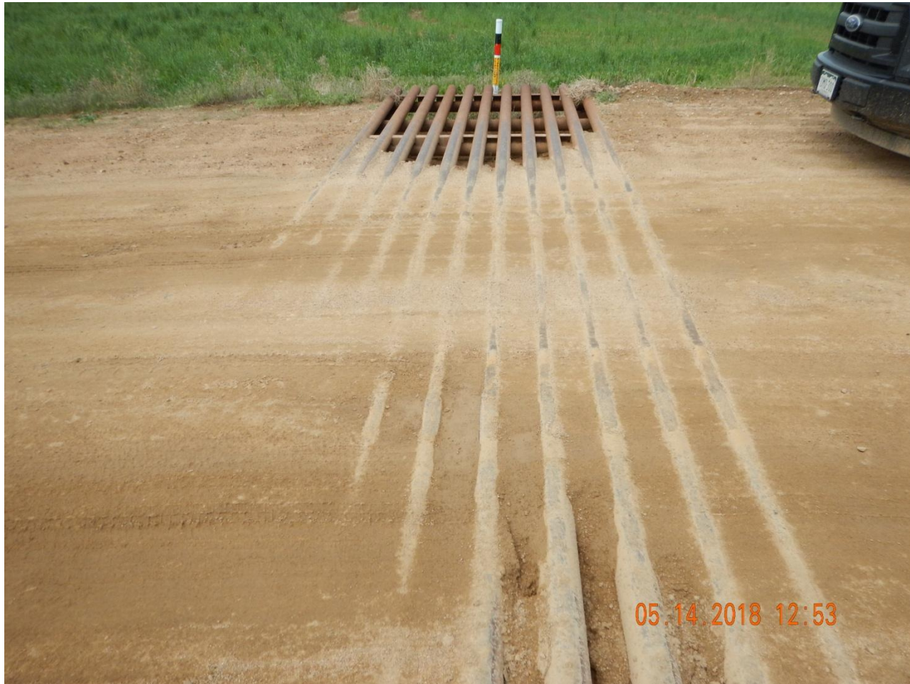
Photo 12. Photo taken from a portion of the access road. Cattle guard in need of maintenance. A similar inspection will be sent to the other Operator that also uses this BMP and access road. Both Operator's will need to coordinate to perform the required maintenance for this BMP.
