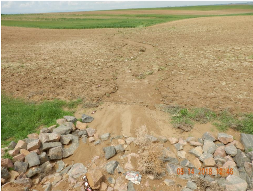
Photo 10. Photo taken from a portion of the access road, facing North. Approximate location in lat/long (40.277356, -104.973795). Rill erosion evident beyond the outlet protection of the culvert. Outlet protection in need of maintenance.
