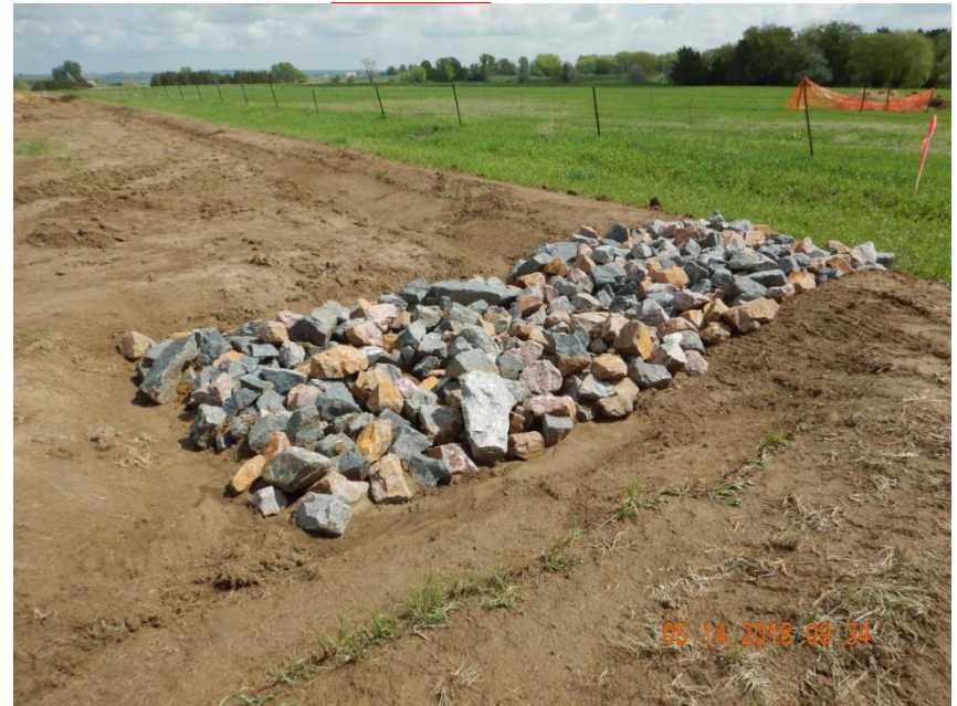
Photo 6. Photo taken from the southeast perimeter of the location, facing North. Rip-rap has been installed in conjunction with the ditch and berm BMP. This would not be considered a sediment trap.
