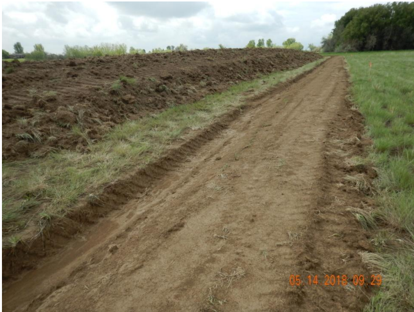
Photo 5. Photo taken from the western perimeter of the location, facing South. Ditch and berm has been installed around the perimeter of the location. Topsoil has been stockpiled along the western perimeter. Does not appear the Operator has salvaged all the topsoil from the location.
