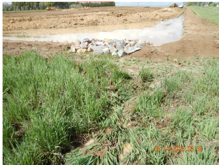
Photo 9. Photo taken from the northwest perimeter of the location, facing West. See comments under Photo 8. Photo illustrates sediment laden discharge actively discharging off location.
