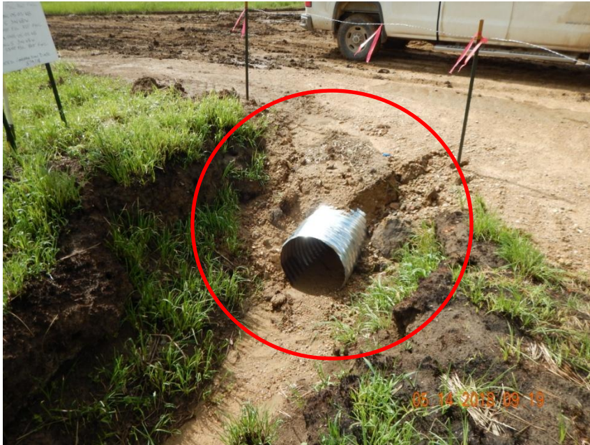
Photo 3. Photo taken from the entrance of the location at culvert #1, facing South. Culverts have been installed along the roadside ditch. Operator needs to stabilize around the culvert to minimize erosion and install inlet/outlet protection.
