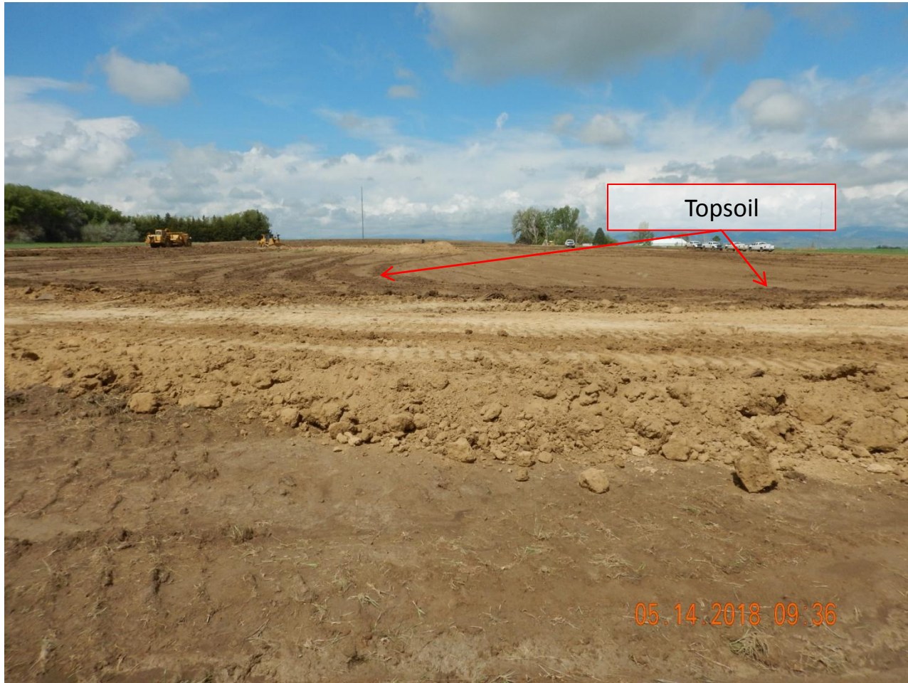
Photo 7. Photo taken from the eastern perimeter of the location, facing North. Based off field observations, Operator has failed to salvage all the topsoil from the location.
