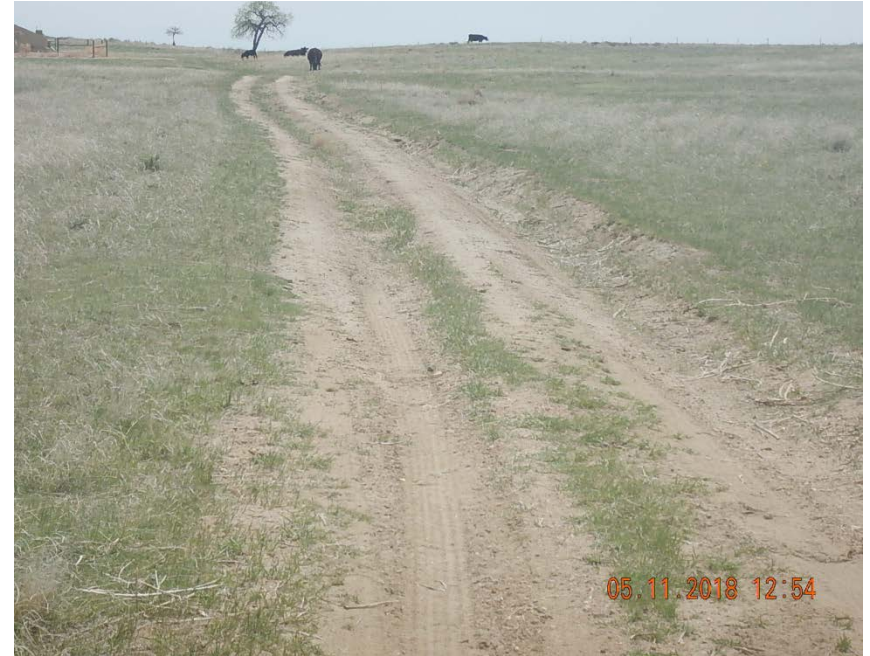
Photo 4: Stormwater rutting on lease road to pump jack, looking S.
