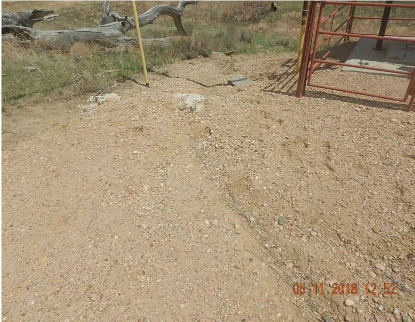
Photo 3: Stormwater erosion on NE corner of location
