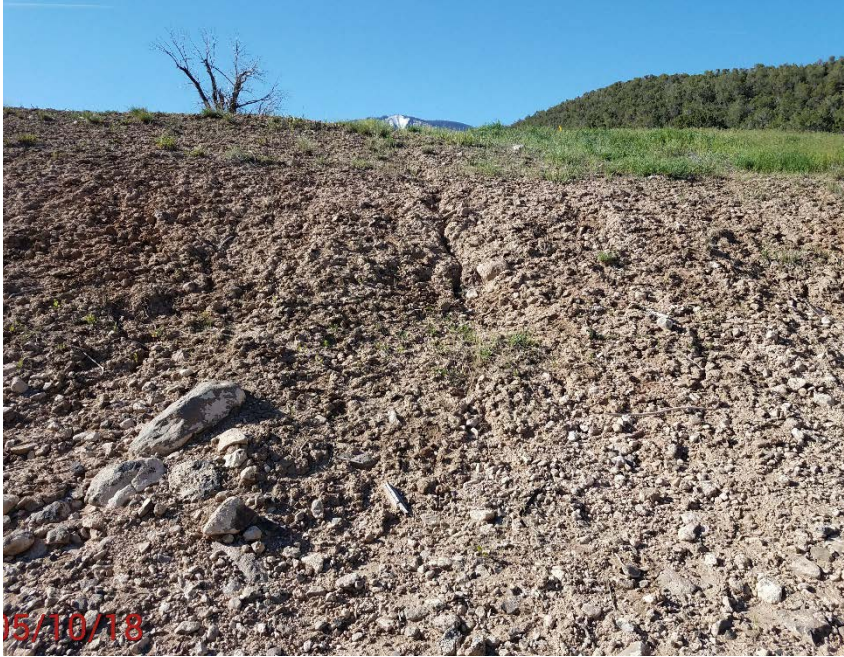
Location photo # 5, Slope erosion on south end of tank battery.
