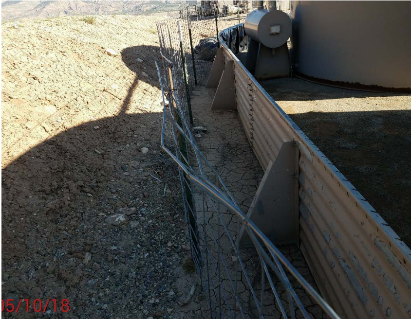
Location photo # 7, Slope erosion on south end of tank battery.
