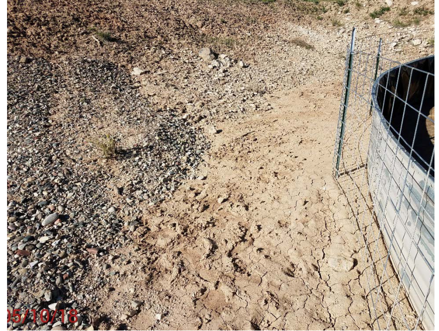
Location photo # 6, Slope erosion on south end of tank battery.
