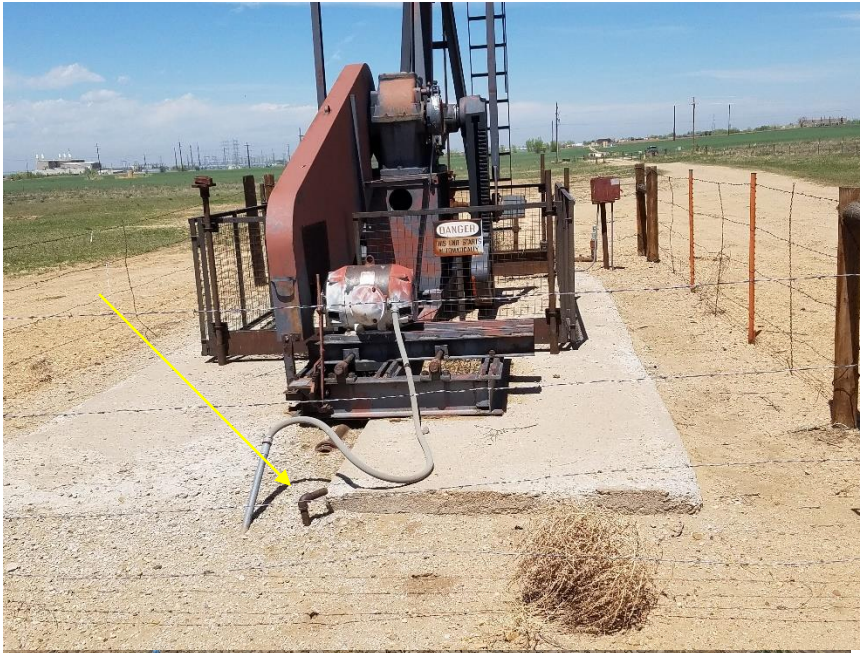
Photo 3. Unmarked riser w/ no LO/TO
