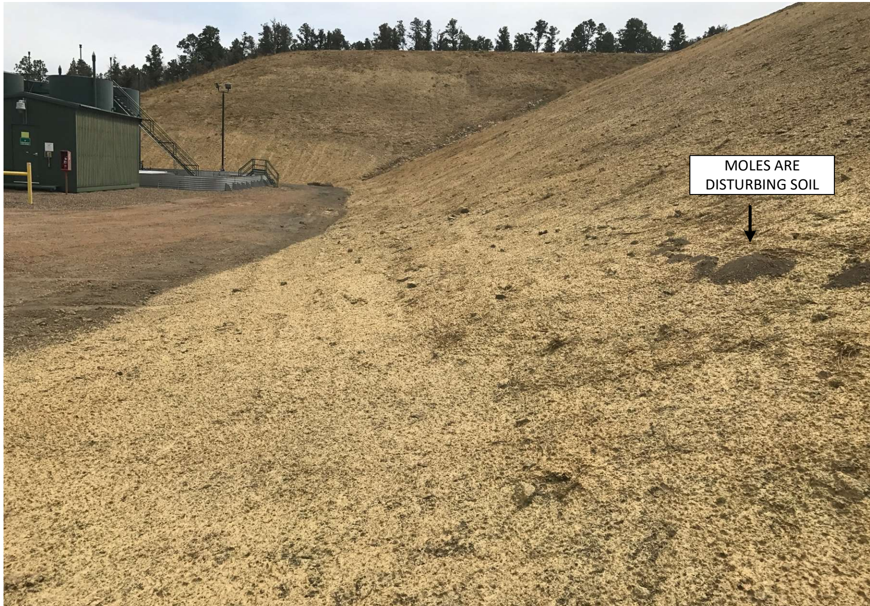
PHOTO 1: OVERVIEW OF LOCATION TO SOUTH. GRADING TECHNIQUES WERE INSTALLED ON THE CONTOUR TO ELIMINATE THE RILL FORMATION ON THE CUT SLOPE. THE EARTH DISTURBANCE WAS STABILIZED BY HYDRO-SEEDING USING AN APPROVED HILL RANCH SEED MIX TO PROMOTE THE ESTABLISHMENT OF VEGETATION.
