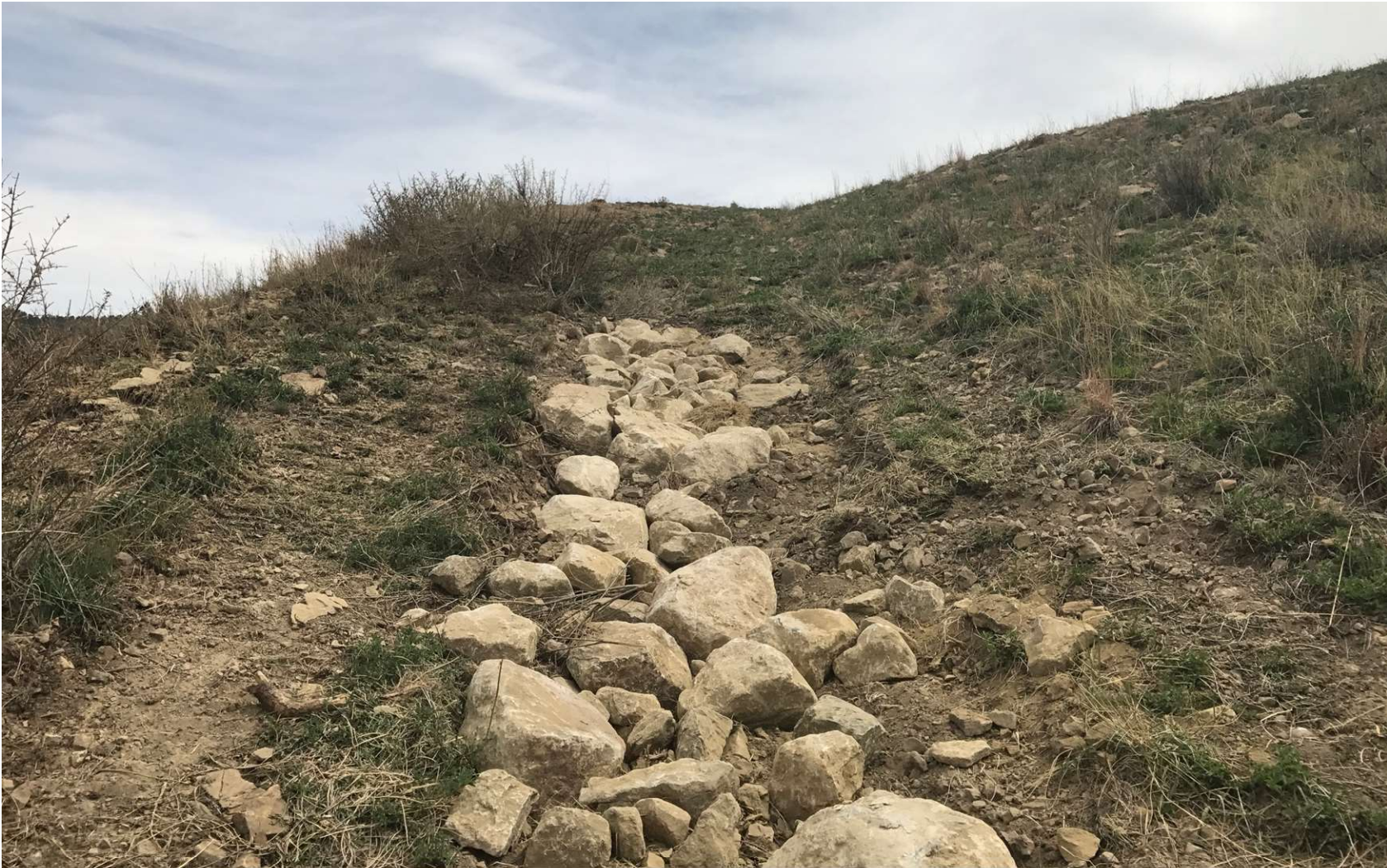
PHOTO 6: RIP RAP WAS PLACED IN THE PORTION OF THE TERRACED SLOPE THAT WAS ERODING TO CONTROL THE EROSION.
