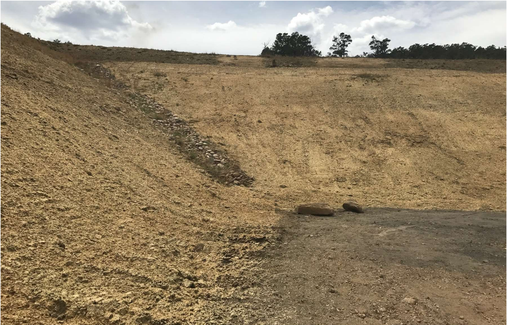
PHOTO 5: GRADING TECHNIQUES WERE INSTALLED ON THE CONTOUR TO CORRECT RILL FORMATION. THE EARTH DISTURBANCE WAS STABILIZED BY HYDRO-SEEDING USING AN APPROVED HILL RANCH SEED MIX TO PROMOTE THE ESTABLISHMENT OF VEGETATION.
