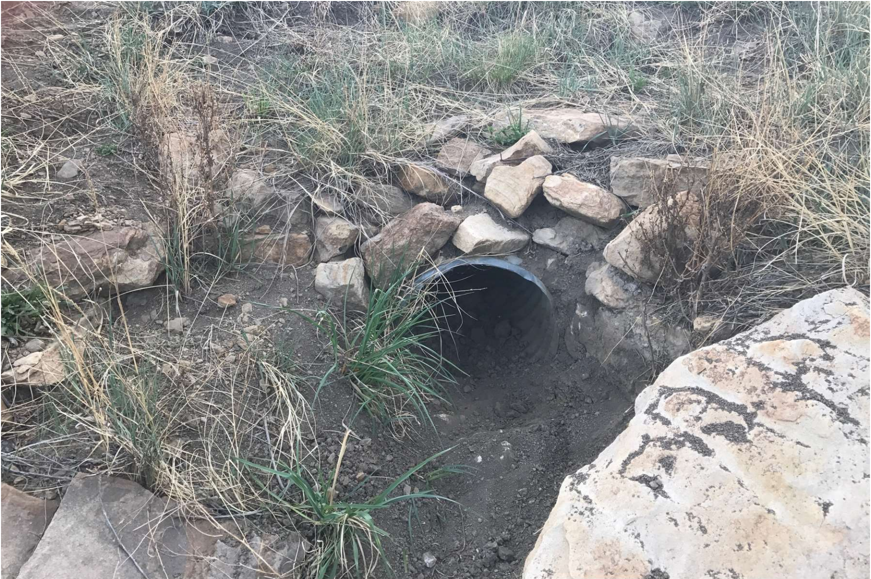
PHOTO 7: THE LOOSE SOIL WAS REMOVED FROM THE CULVERT OUTLET.
