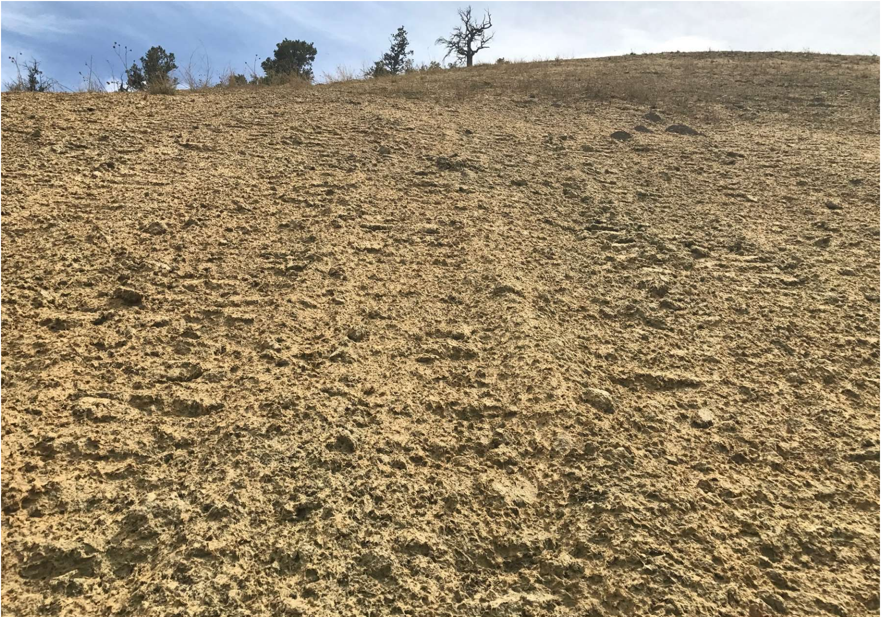
PHOTO 4: GRADING TECHNIQUES WHERE INSTALLED TO REMOVE RILL FORMATION.
