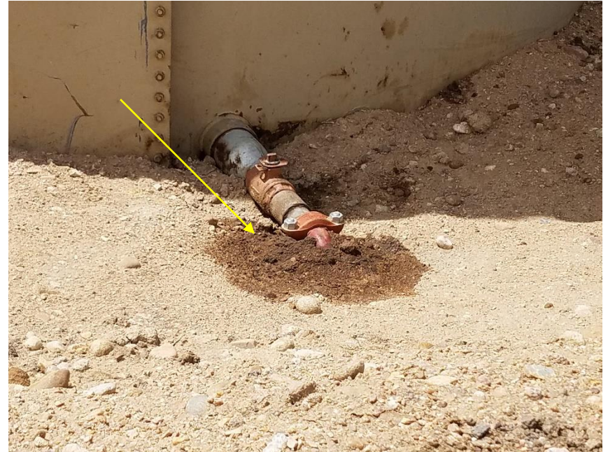
Photo 6. Stained soil near outlet of tank
