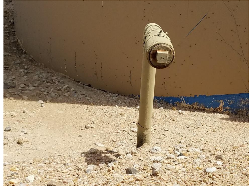
Photo 8. Unmarked riser on east side of crude oil tanks
