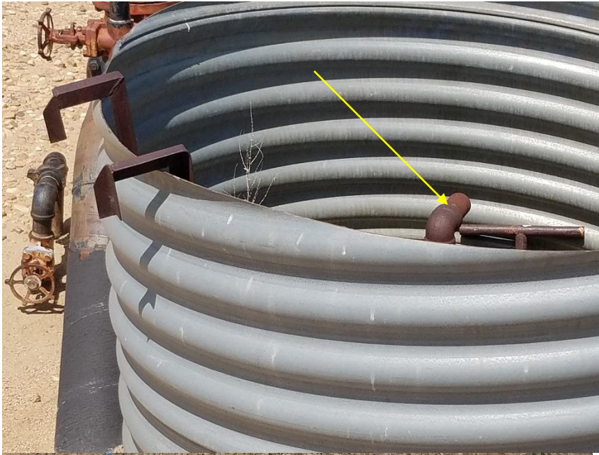
Photo 9. 2 unmarked risers inside containment near meter house, second riser is not visible in picture.
