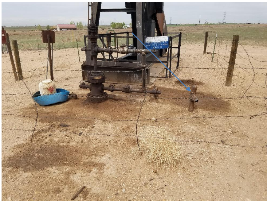
Photo 1. Wellhead/stained soil, unmarked riser No LO/TO.
