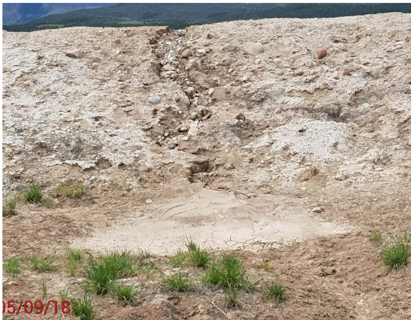
Location photo # 5, slope erosion near retention pond
