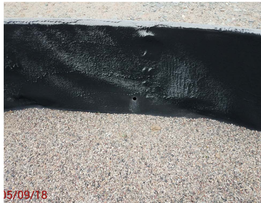
Location photo # 6, Hole in containmnet
