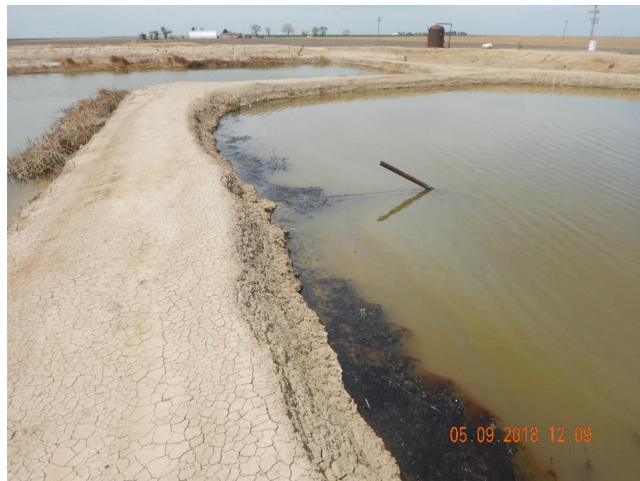
Photo 4: Photo taken from the south end, of the north-central produced water pit. Photo shows hydrocarbons in the produced water pit.
