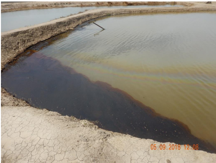
Photo 3: Photo taken from the southeast corner, of the north-central produced water pit. Photo shows hydrocarbons in the produced water pit.
