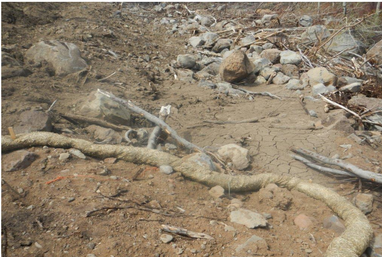
Photo#18: Ineffective BMP at base of fill slope.
