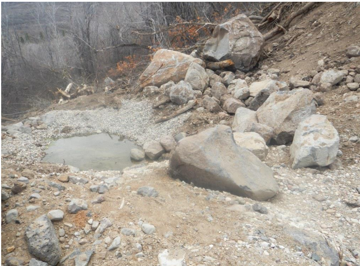
Photo#5: Sediment trap receiving flow from french drain routing Spring water. View to East.
