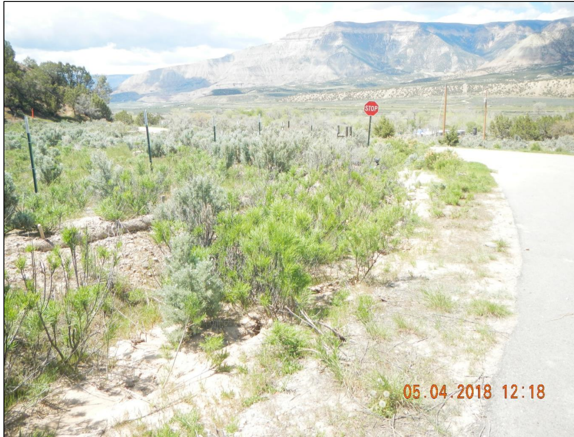
Sediment build up in ditch at county road and access road intersection.
