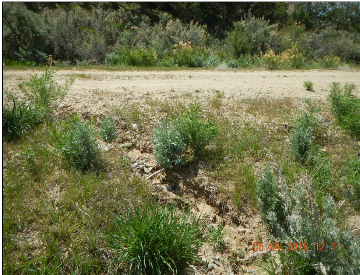
Erosion rill on road side.
