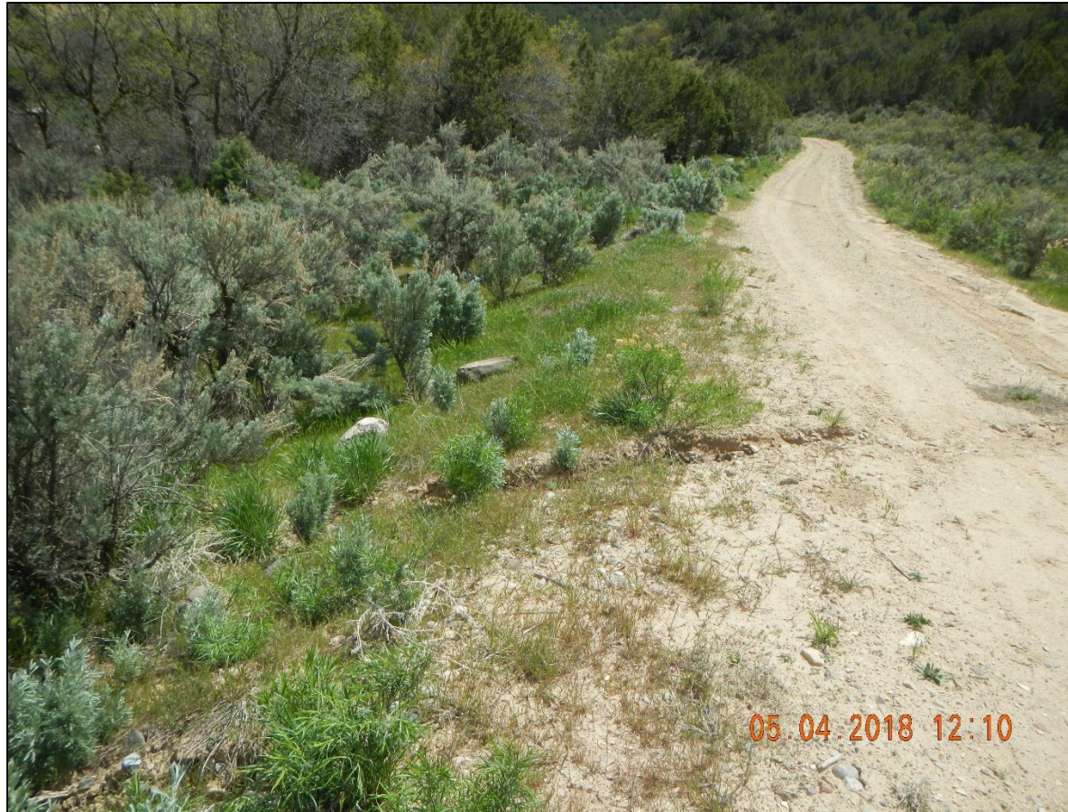
Erosion rill on road side.
