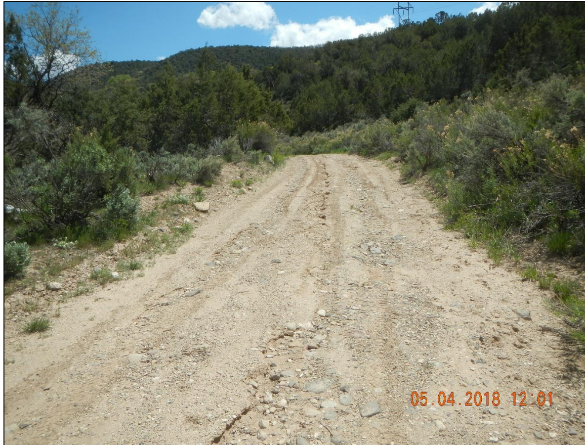
Ruts moving sediment and erosion on access road. Looking up hill.
