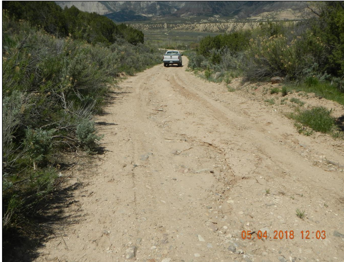
Ruts moving sediment and erosion on access road. Looking down hill.
