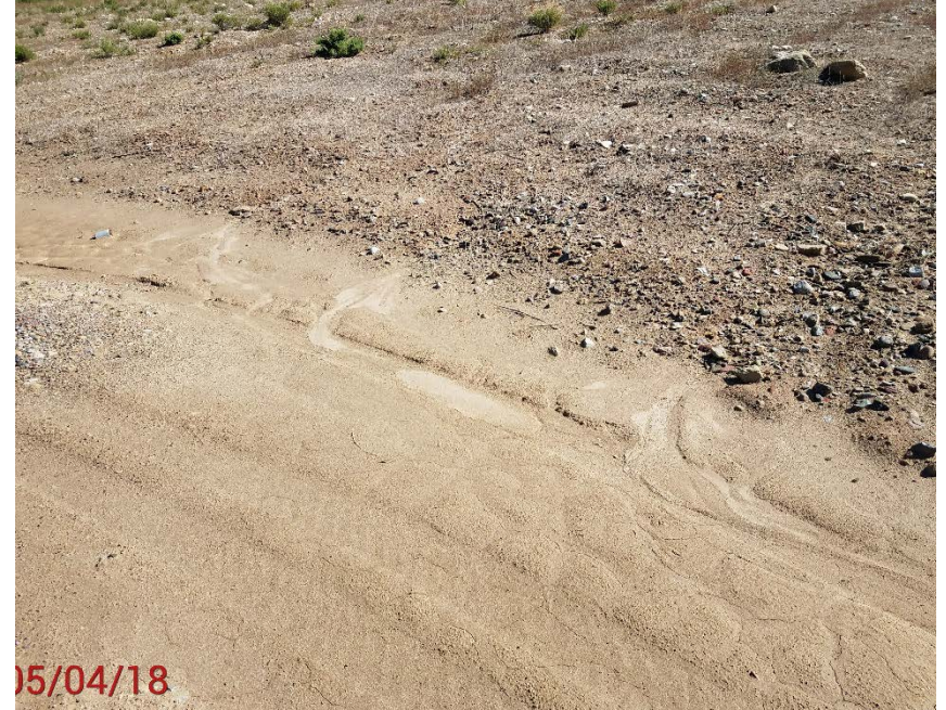
Location photo # 6, Slope erosion East end of location
