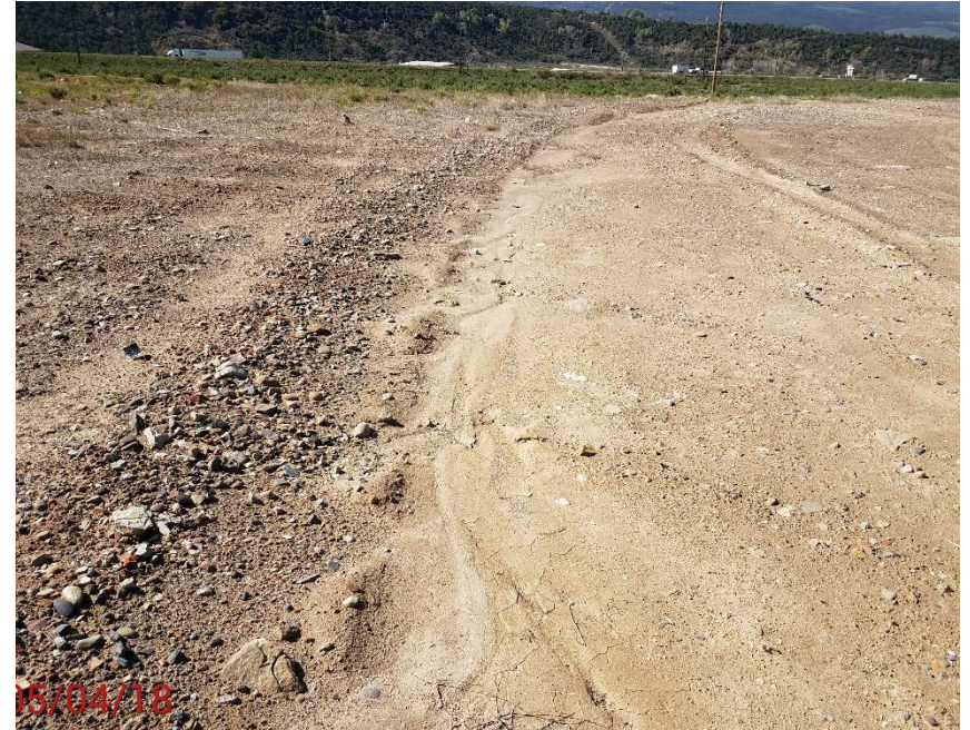
Location photo #8, Slope erosion East end of location
