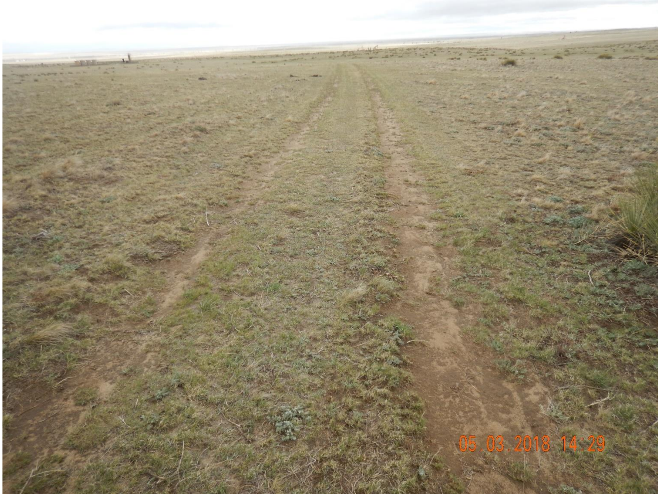
Photo 7: Photo taken from the access road, facing east. Photo shows sections of access road where vegetation does not appear to be establishing. Additional revegetation activities may be required.
