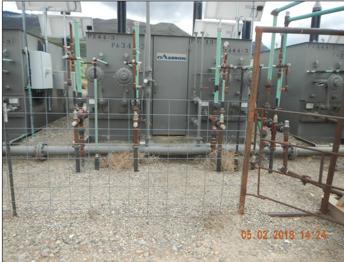
Weed debris around separators.
