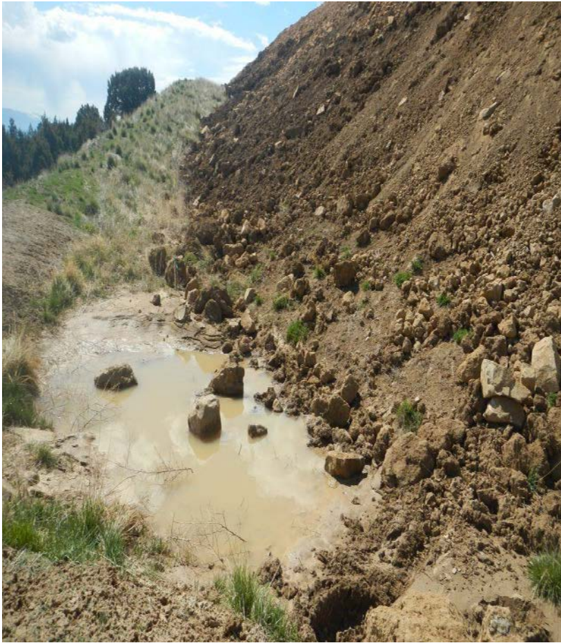
Photo#2: Sediment trap at base of fill slope. View to South
