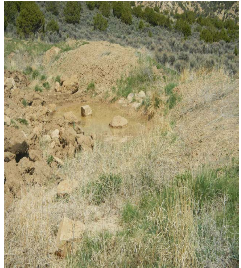
Photo #3: Sediment trap at base of fill slope. View to North
