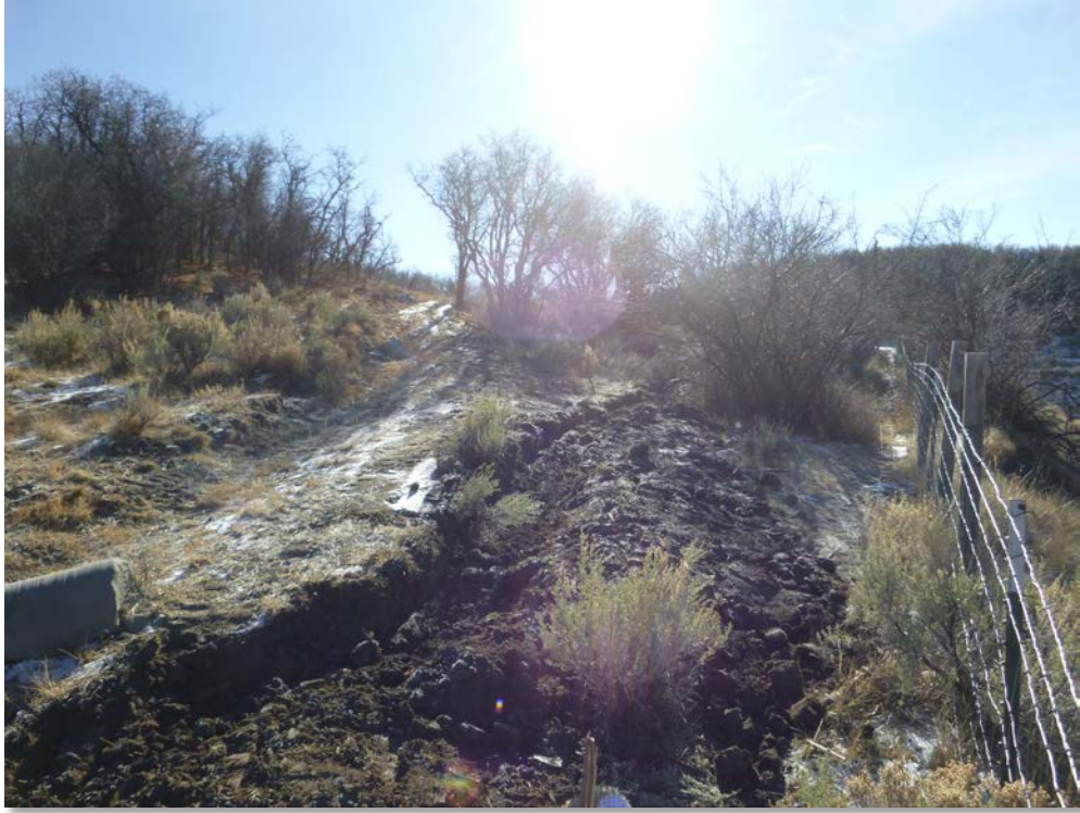
Photo 1. Installation of an additional Diversion Ditch above the Cut Slope as recommended by COGCC.
