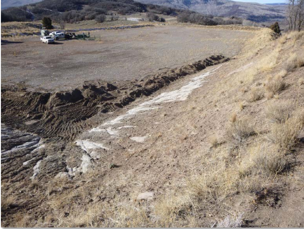
Photo 3. Deepening of on-pad Diversion Ditch to prepare for installation of Jute Matting in Spring 2018.
