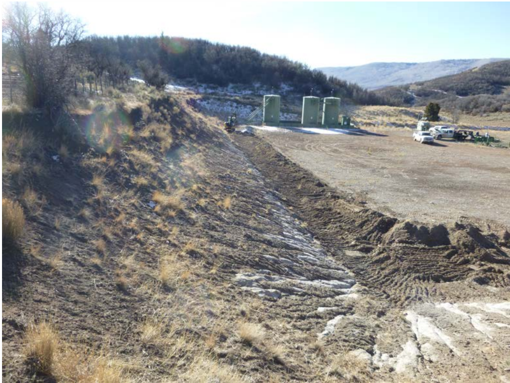
Photo 2. Deepening of on-pad Diversion Ditch to prepare for Jute Matting Installation in Spring 2018.
