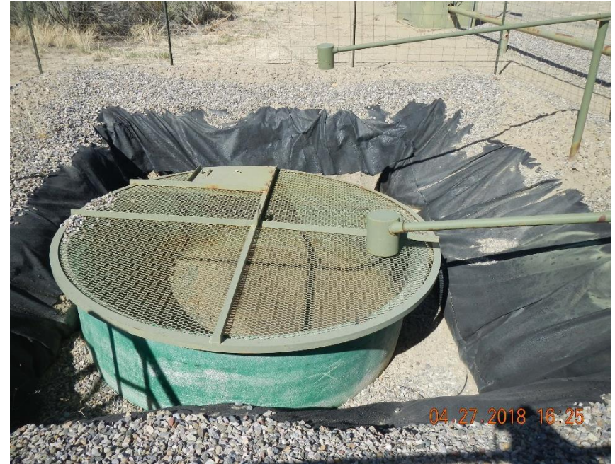
Fiberglass open topped 20 bbl. tank.
