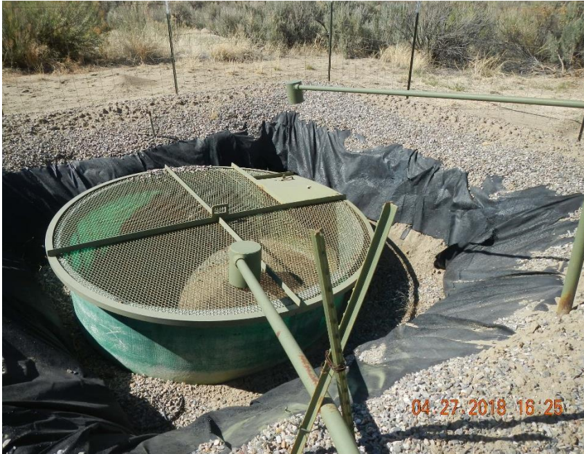
Gravel berm has sloughed off into containment area. Liner is torn.
