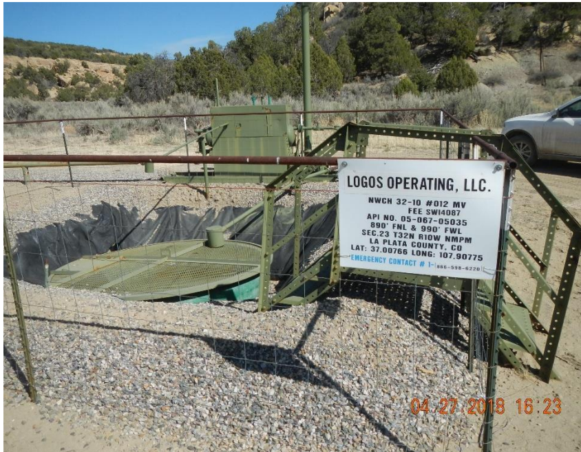
Location sign and fiberglass open topped tank.
