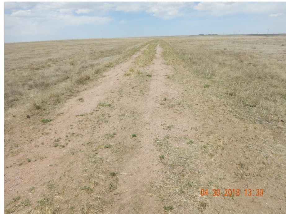
Photo 11: Photo taken from the sign seen in photo 10 within the access road. Photo shows remaining section of access road to the north. Photo shows no reclamation activities appear to have been performed; gravel remains on road, access road has not been re-contoured, re-graded or had compaction alleviation conducted. Operator remains responsible for reclamation of access road.
