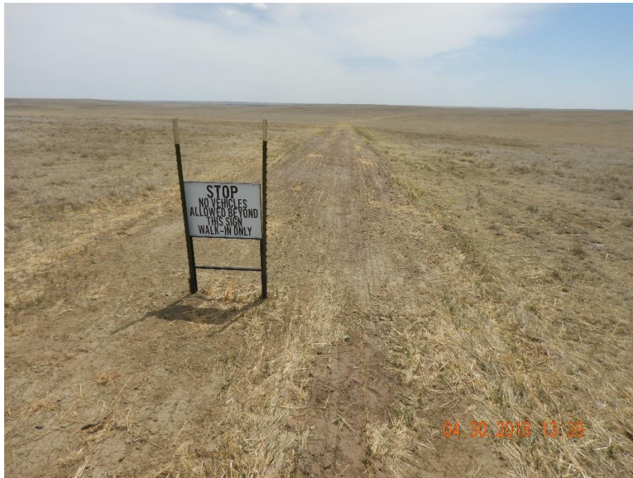
Photo 10: Photo taken from the access road to the north of the location. Photo shows sign where operator appears to have ended reclamation of the access road. Access road continues ~1/4 mile to the north. Operator remains responsible for the reclamation of these areas of access road.
