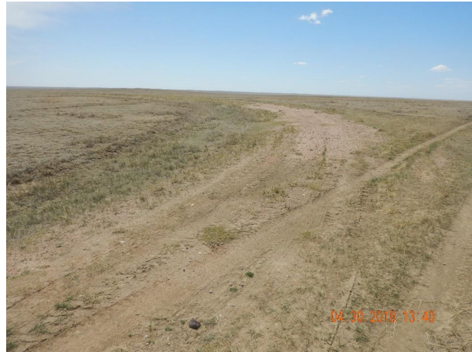
Photo 12: Photo taken from the area where the access road joins the east/west ranch road, north of the sign seen in photo 10, facing southwest. Photo shows remaining section of access road where no reclamation activities appear to have been performed; gravel remains on road, access road has not been re-contoured, re-graded or had compaction alleviation conducted. Operator remains responsible for reclamation of access road.
