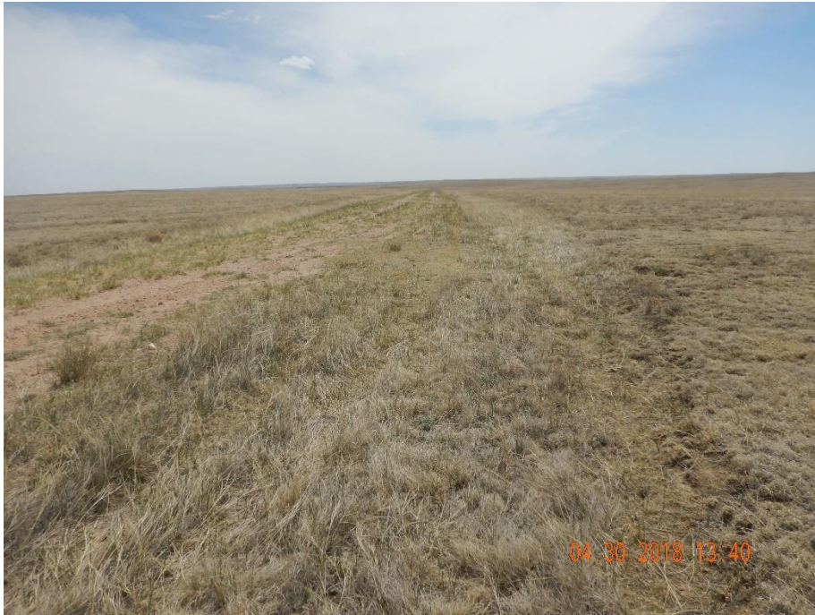
Photo 11: Photo taken from the area where the access road joins the east/west ranch road, north of the sign seen in photo 10, facing south. Photo shows remaining section of access road where no reclamation activities appear to have been performed; gravel remains on road, access road has not been re-contoured, re-graded or had compaction alleviation conducted. Operator remains responsible for reclamation of access road.
