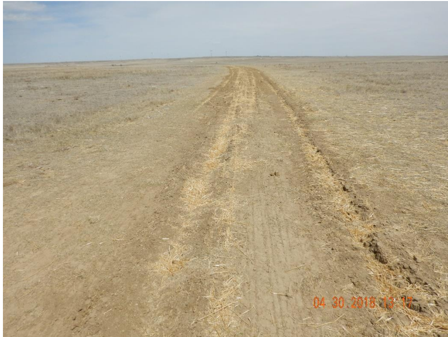
Photo 5: Photo taken from the access road entrance, facing northeast. Photo shows additional work appears to have been conducted, however, it also appears a two-pronged ripper only cut through areas of the ruts within the road. Compaction alleviation does not appear to have conducted in accordance to reclamation requirements. Compaction concerns remain on access road.
