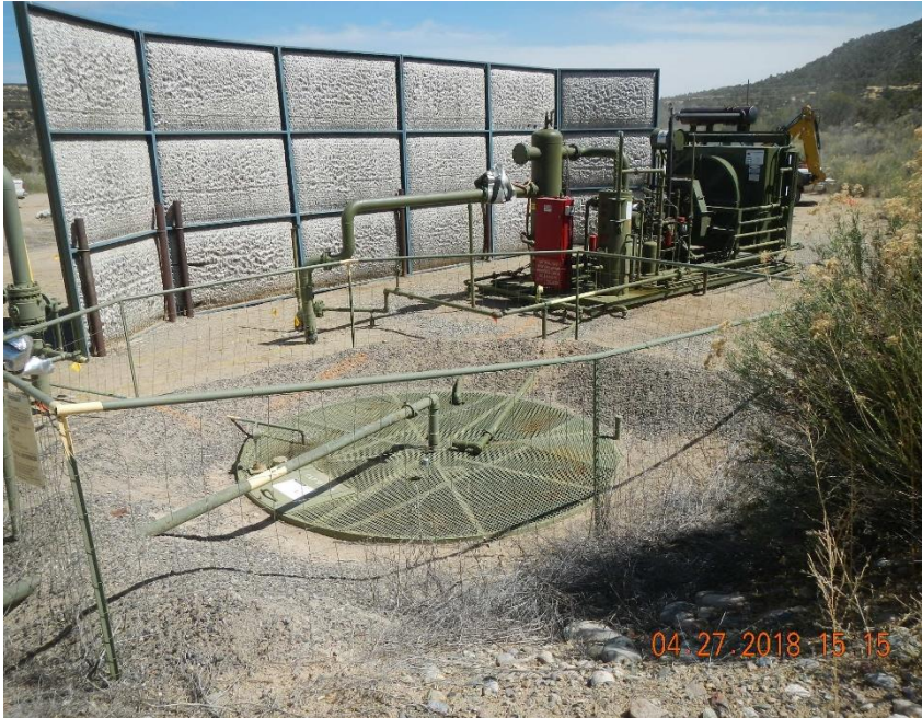
PBV and skid mounted compressor.
