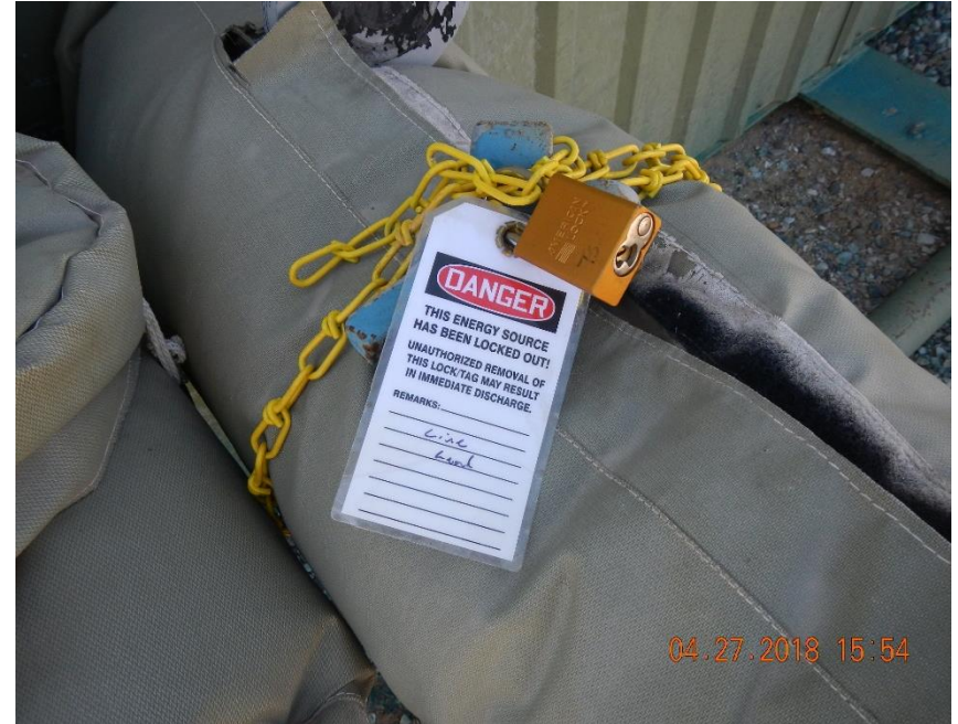
Locked out valve at Hendrickson Water Injection Facility.
