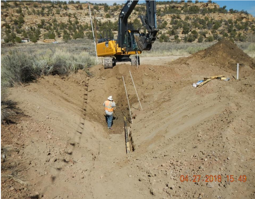
Excavation of 4" steel produced water line.
