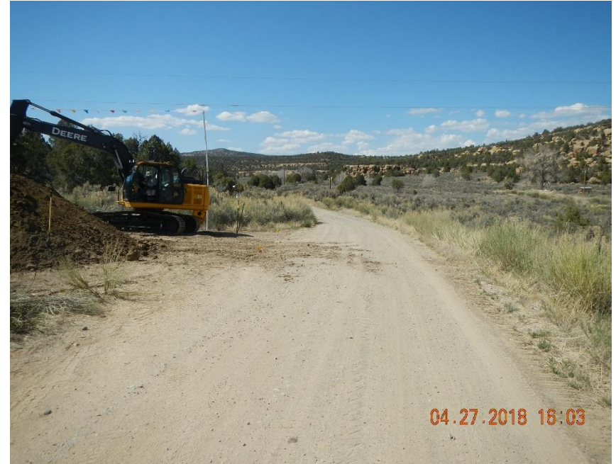
Track hoe excavating 4" water transfer line.
