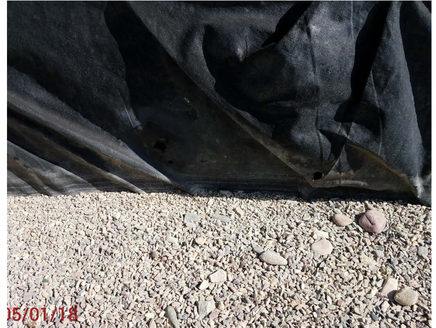
Location photo #6, Holes in tank battery containment
