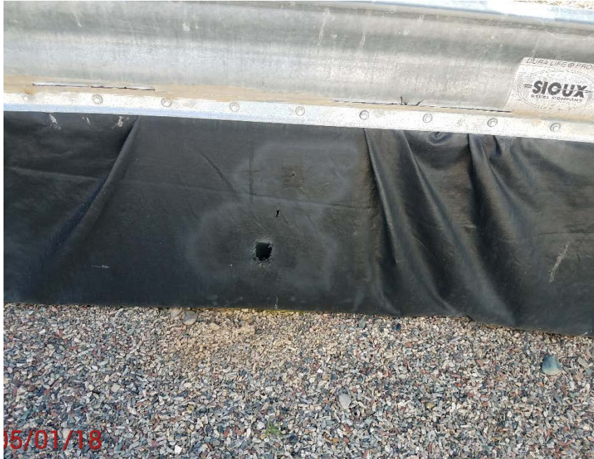
Location photo # 9, Holes in tank battery containment
