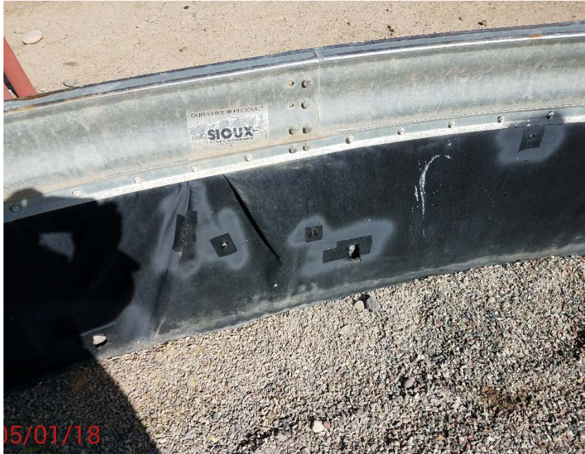
Location photo # 7, Holes in tank battery containment
