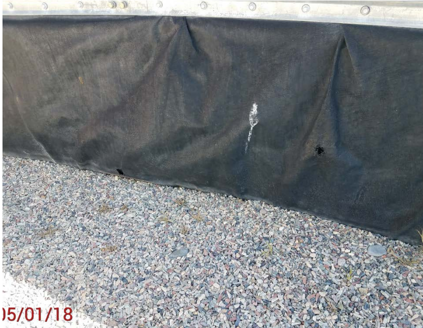
Location photo # 5, Holes in tank battery containment
