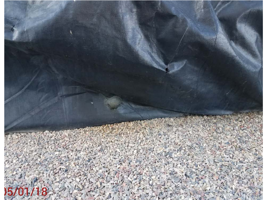
Location photo #8, Holes in tank battery containment
