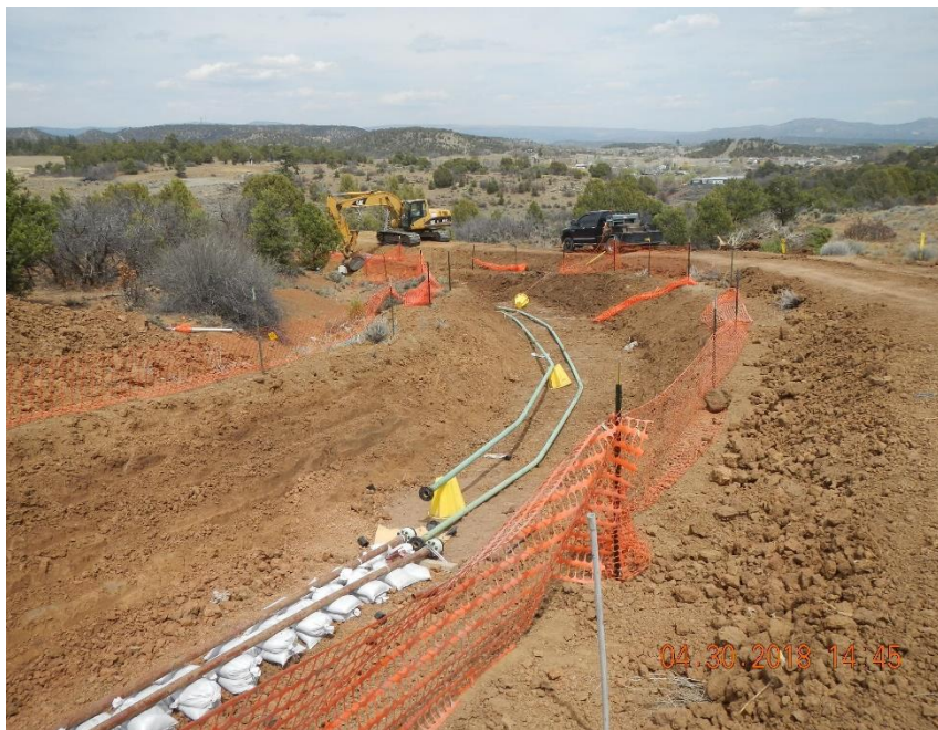
New section of steel pipe in area where failure occurred.
