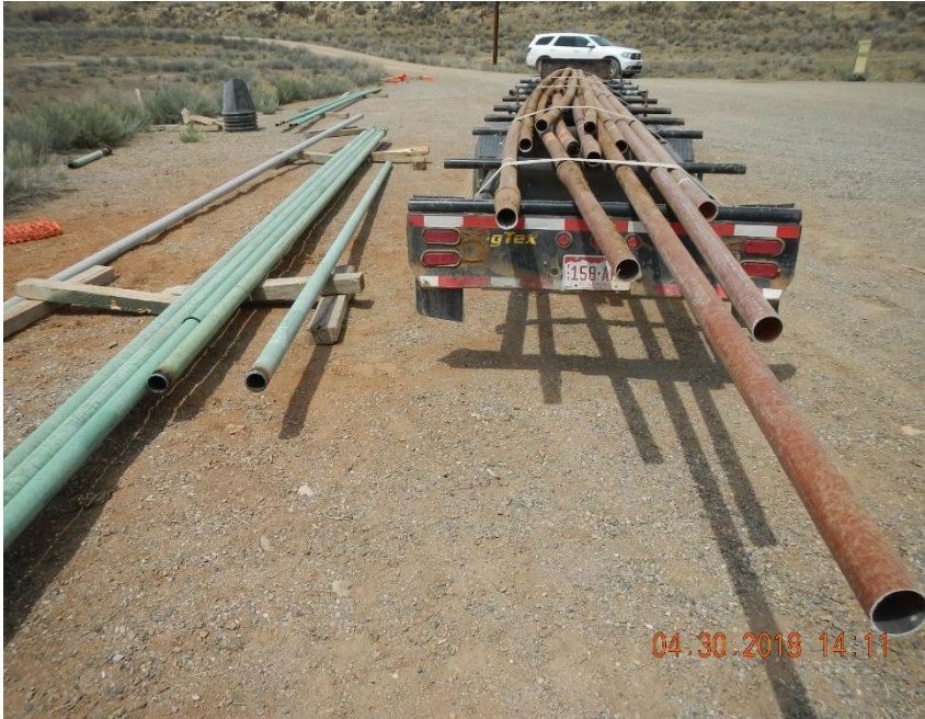
Sections of 3" fiberglass pipe being replaced with steel pipe.
