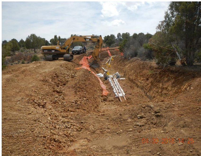
New sections of steel pipe being installed.
