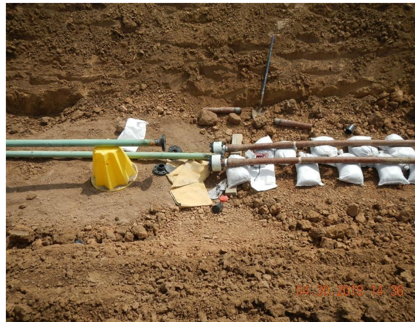
Transition from fiberglass pipe to new steel pipe.
