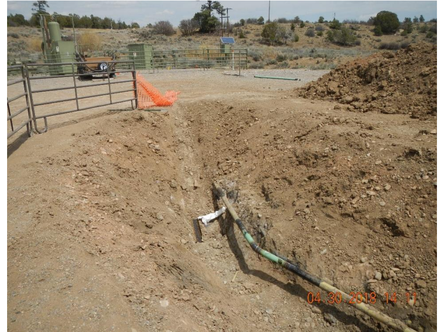
Repaired section of transfer line on location.
