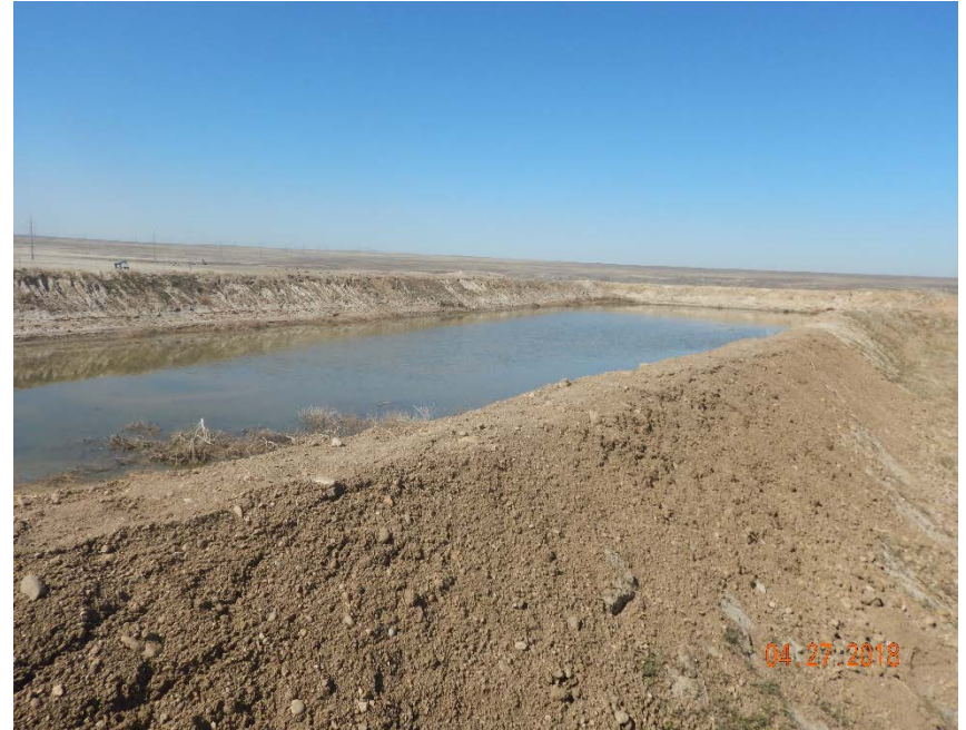
Photo #12 – View looking SW over evaporation pit documents berm repair and weed control efforts.
