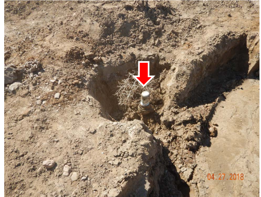
Photo #6 – Flowline riser at SE corner of former produced water AST location.
