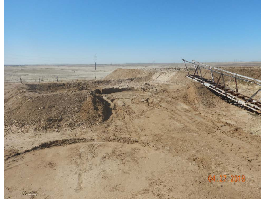
Photo #4 – 300 bbl produced water AST has been removed, additional work required to remove unused equipment and to reclaim former earthen berm.
