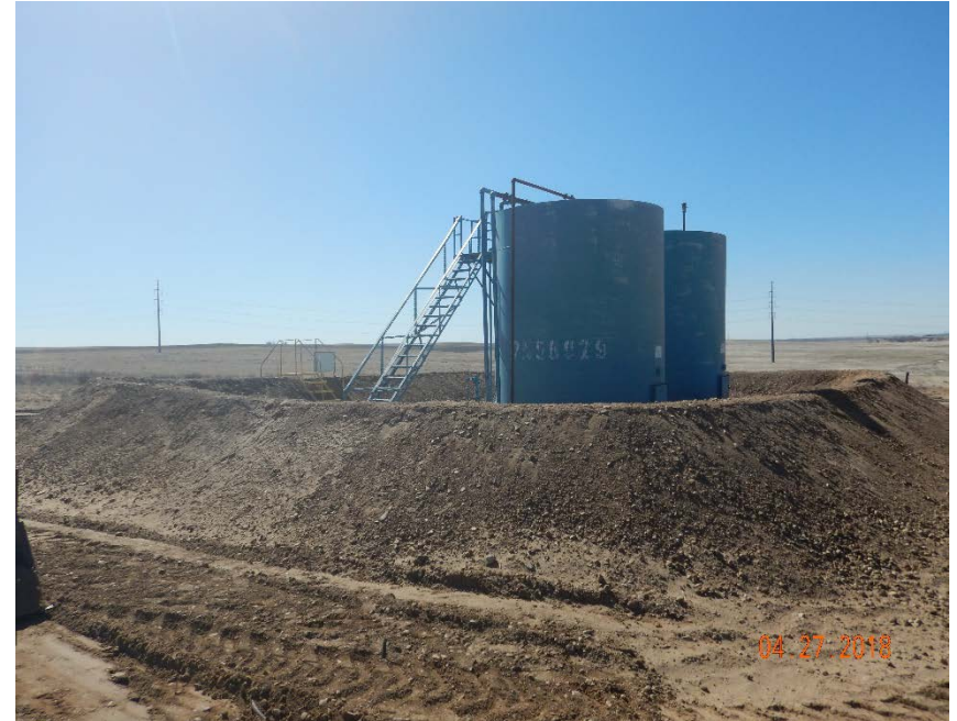
Photo #2 – View from NW of tank battery documents that operator has improved berms on location.
