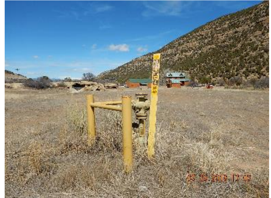
Photo 10: E side riser with steel post and pole barrier.
