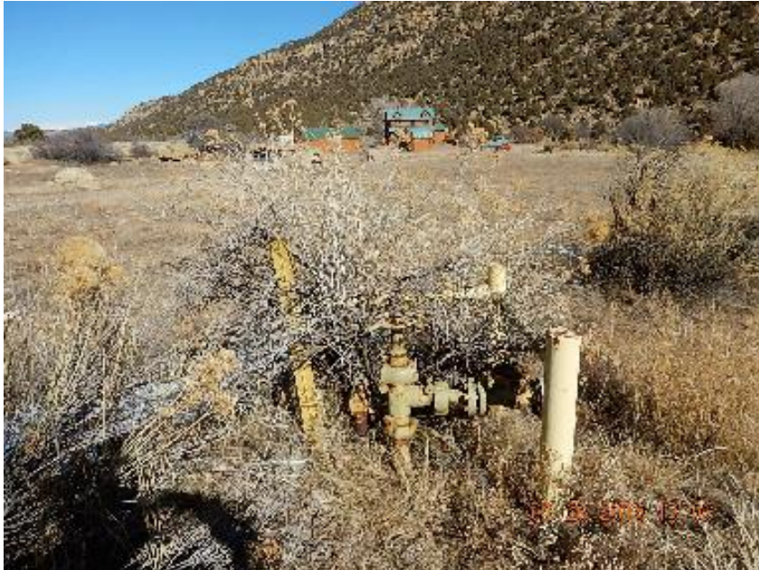
Photo 5: W side (2) risers with steel post and pole barrier. Previous inspection.
