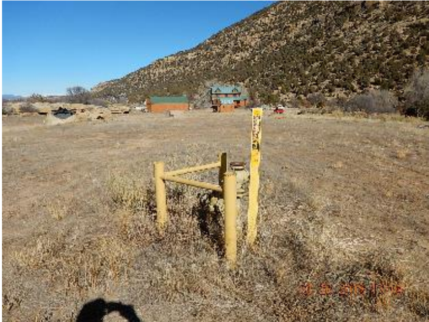
Photo 9: E side riser with steel post and pole barrier. Previous inspection.
