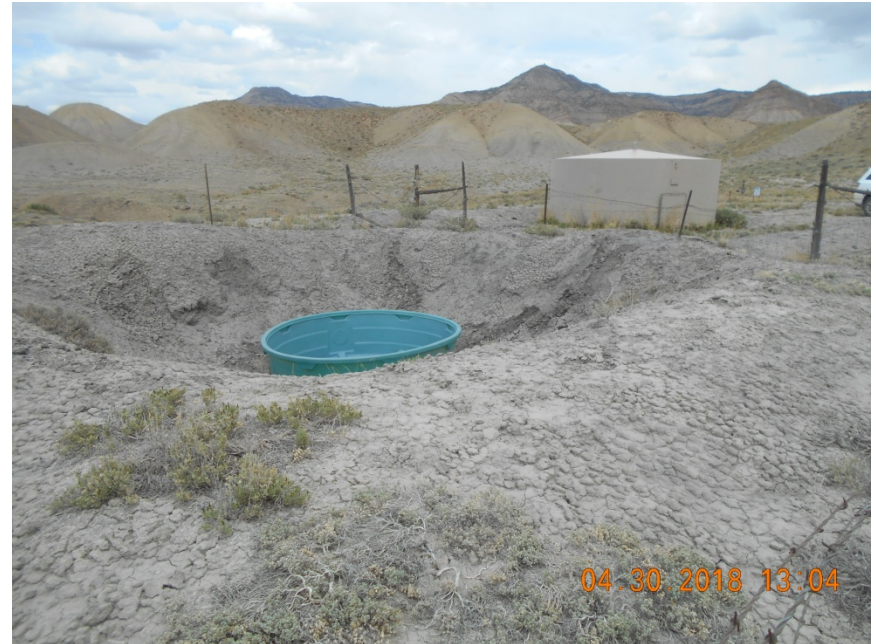
Blowdown pit with plastic tank on S. side of location
