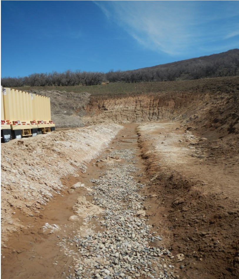
Photo#2: View to NE of eroding cut slope.
