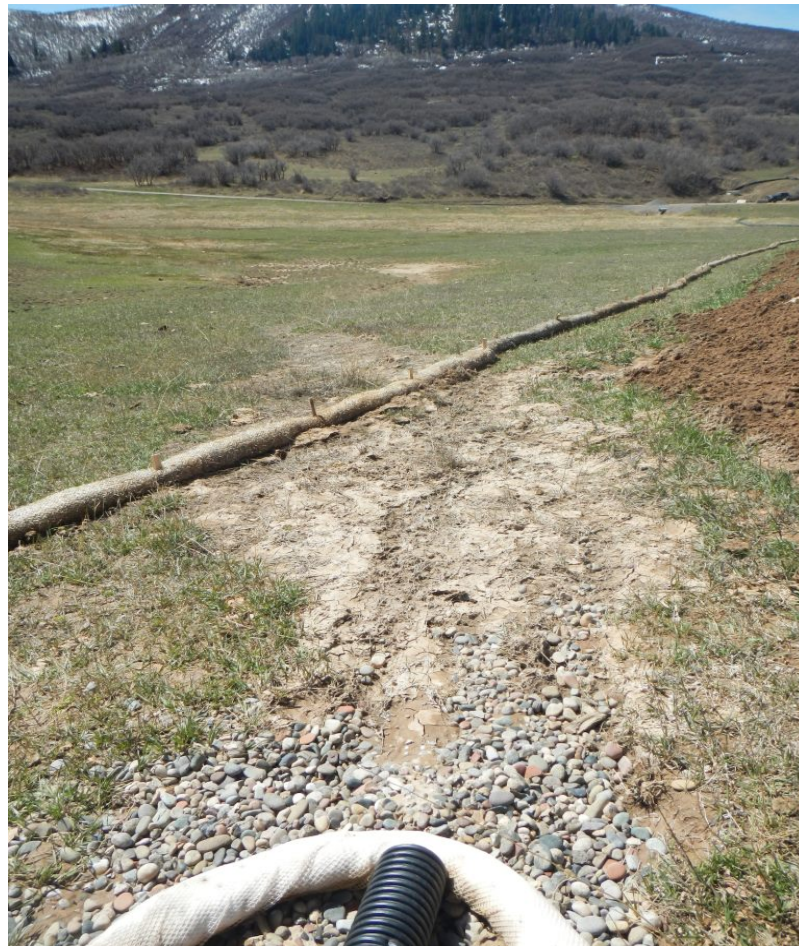
Photo#5: BMP outlet / discharge leading from eroding cut slope, showing sediment migration.. April 18, 2018
