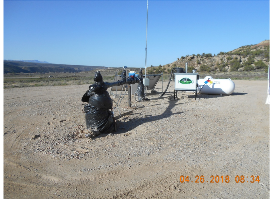
Wellhead with line heater.
