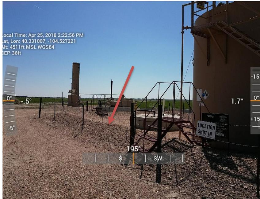
**Berm are worn down around tanks and separator.**
