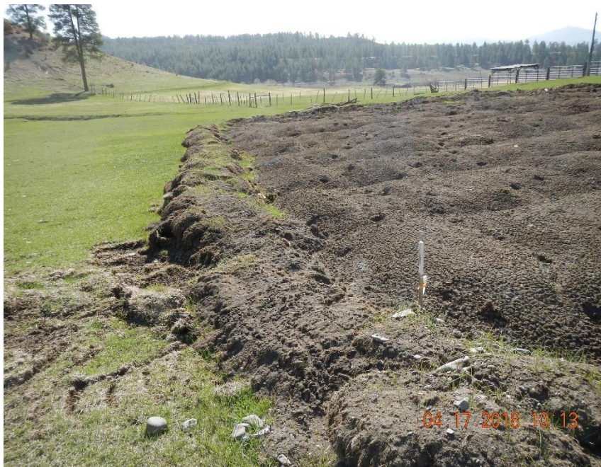
Containment berm along northern edge of land farm treatment cell.
