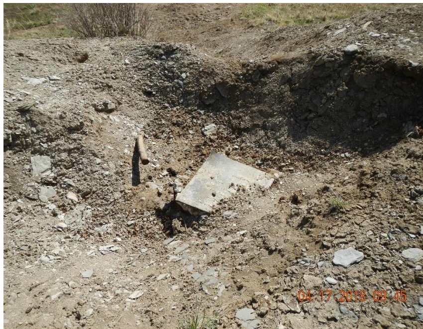
Fitzhugh #15 PA marker and abandoned flow line.
