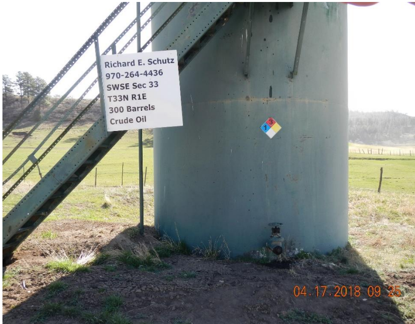
Crude oil AST without secondary containment.
