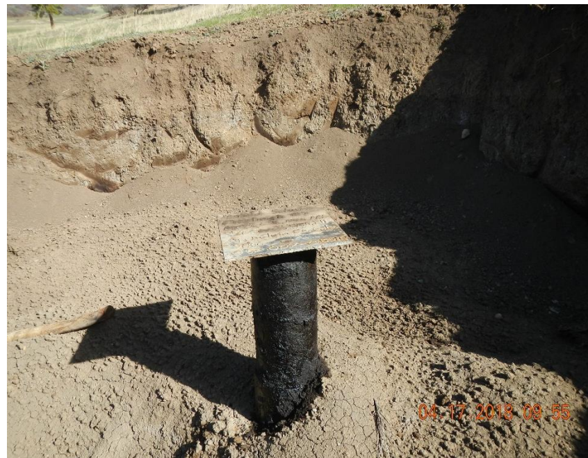
Fitzhugh #7 casing is stained with oil.
