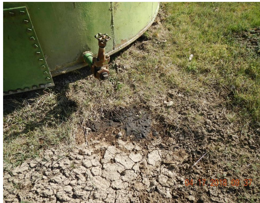
Stained soil beneath load out valve on unused AST.
