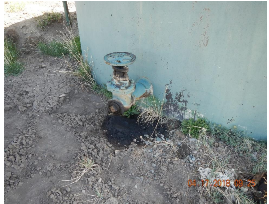
Stained soil beneath load out valve.
