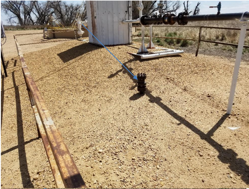
Photo 3. Unmarked riser
