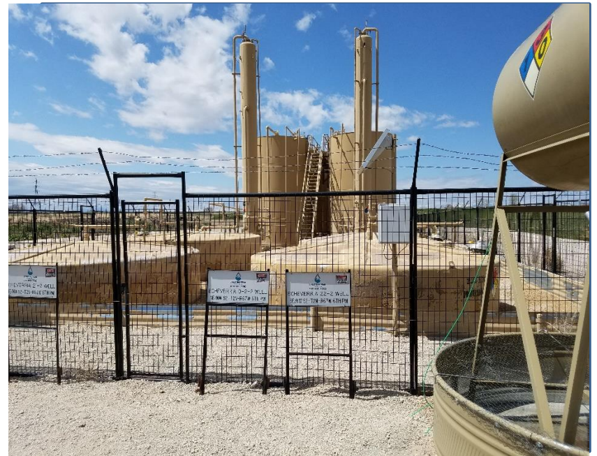
Photo 2. Tank battery
